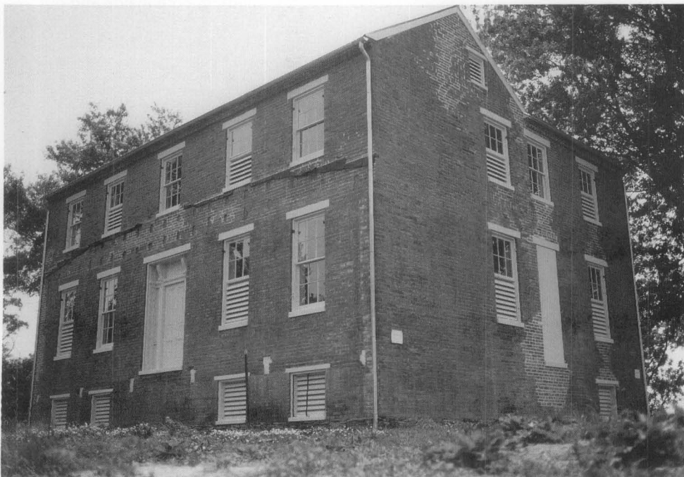
Figure 1. Proper mothballing treatment: This building has been successfully mothballed for 10 years because the roof and walls were repaired and structurally stabilized, ventilation louvers were added, and the property is maintained. Photo: Charles E. Fisher, NPS.
