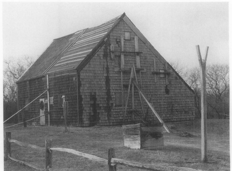
Figure 3. Buildings seriously damaged by storms or deterioration may need to be braced before architectural evaluations can be made. Jethro Coffin House. Photo: John Milner Architects.
