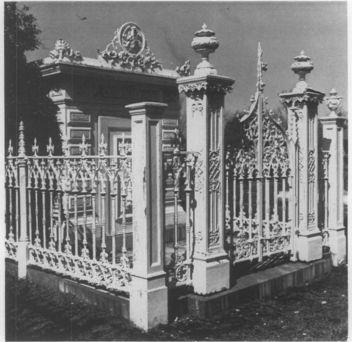
Fig. 5. The Slatter Family Tomb in Mobile, Alabama, consisting of a cast-iron mausoleum and fence, exhibits the wide range of uses of the material in the 19th century. Photo: Jack E. Boucher, HABS Collection.
