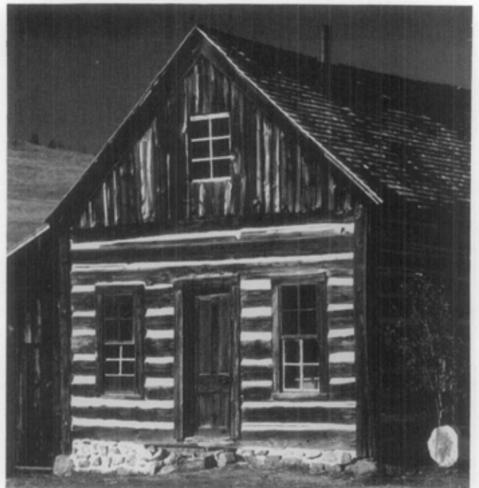
Fig. 9. This historic log building on the Walker Ranch in Boulder, Colorado is an example of the Rocky Mountain cabin form which is typified by the entrance door being located in the gable end. Photo: Bernard Weisgerber.
