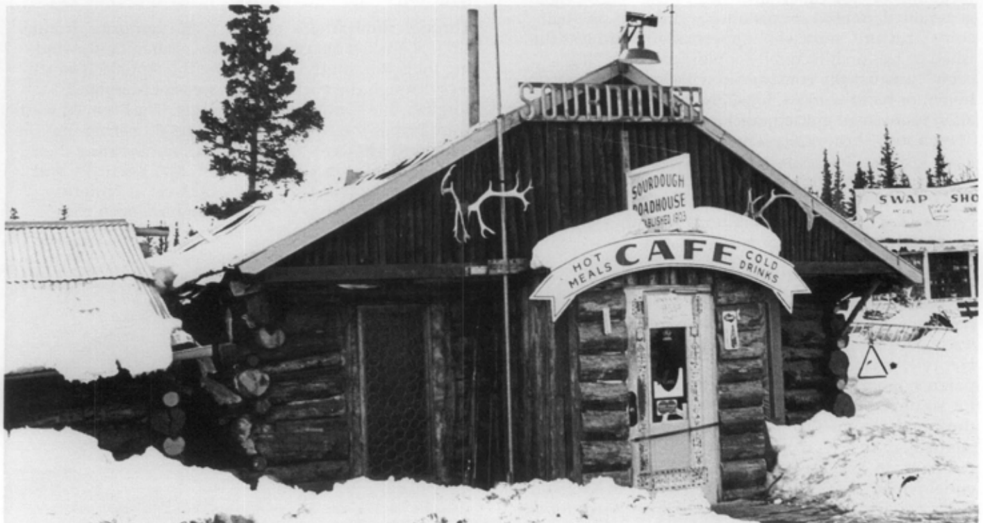
Fig. 1. Log construction was practical in the rough frontier and climate of Alaska, where it was used for a variety of structures such as the Sourdough Lodge (c. 1903) near Gakona. Built to serve the trail leading to the Klondike gold discoveries, this 1-story, L-shaped roadhouse is primarily of horizontal log construction with vertical logs in the front gable. Photo: National Park Service Files.
