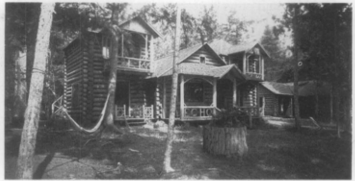
Fig. 5. The main lodge of Echo Camp on Raquette Lake in New York State was built in 1883 by the governor of Connecticut. It typifies the Adirondack style in the use of exposed round logs with crowns, and porches and balconies constructed with bowed logs and round log columns. Photo: Courtesy The Adirondack Museum.
