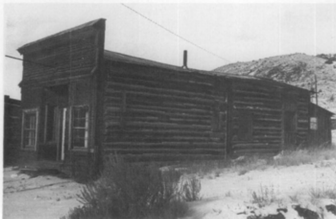
Fig. 4. Beginning around the mid-19th century, entire western boottowns were hastily constructed of frame and log, such as the buildings in Bannack, Montana, the site of the State's first gold discovery. Photo: National Park Service Files.
