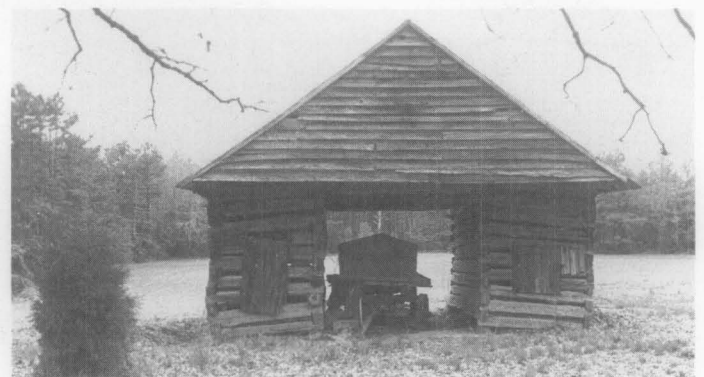
Fig. 3. This mid-19th century double-pen corncrib on the Jamison Farm in Rowan County, North Carolina, is an example of a type of log building that did not require chinking. Photo: Denise Whitley.
