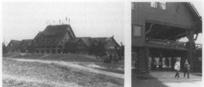
Fig. 6. (a) Old Faithful Inn, Yellowstone National Park, Wyoming, shown here in 1912, brought the Rustic style to the West in 1903 in an original design, and a scale befitting its setting. (b) Although only the first story is of horizontal log construction, the use of logs is striking in the trestle work and cribbed piers around the entrance. Photo: (a) Courtesy National Park Service, (b) Laura Soulliere Harrison.
