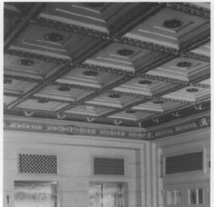
Fig. 9. The elaborate coffered ceiling was designed for the Willard Hotel in Washington, D.C. (1902–04) by Henry Janeway Hardenbergh. The coffered ceiling was restored as part of a rehabilitation project in the 1980s. Photo: Carol M. Highsmith.
