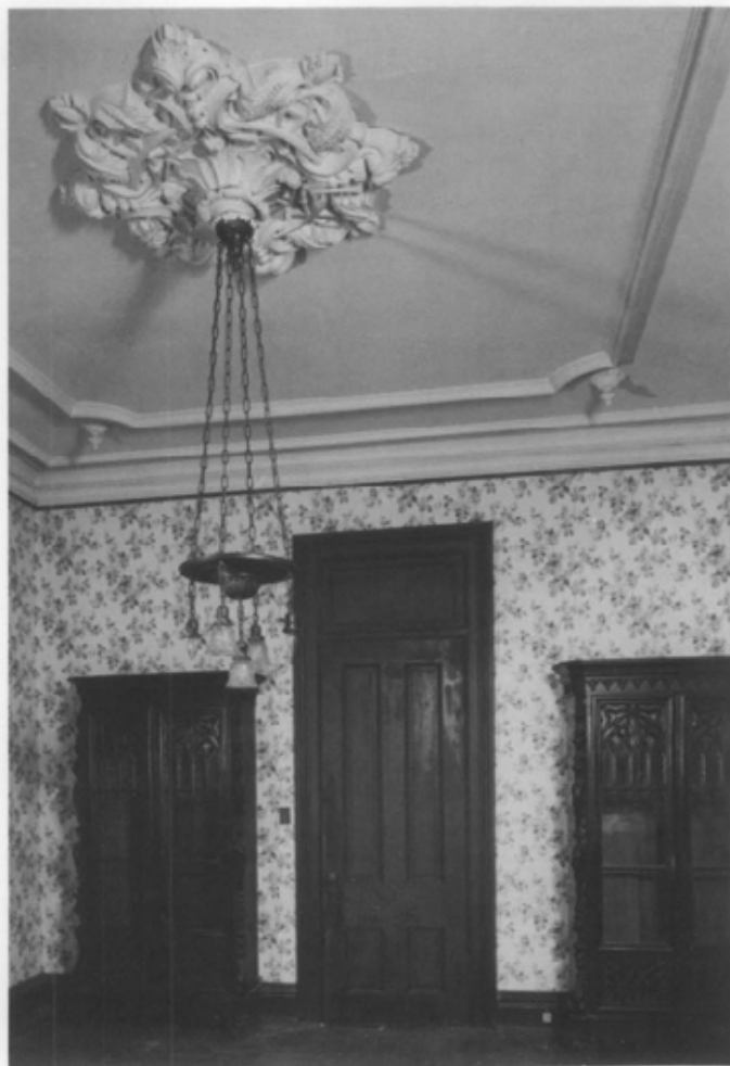
Fig. 2. This parlor medallion and pendant drops shown in a mid-19th century row house in Annapolis, Maryland were originally ordered from a catalog. A local plasterer ran the plain cornice and band ribbon, the curved corners of which were bench run, set with plaster adhesive and pointed at the joints. Photo: M. E. Warren.
