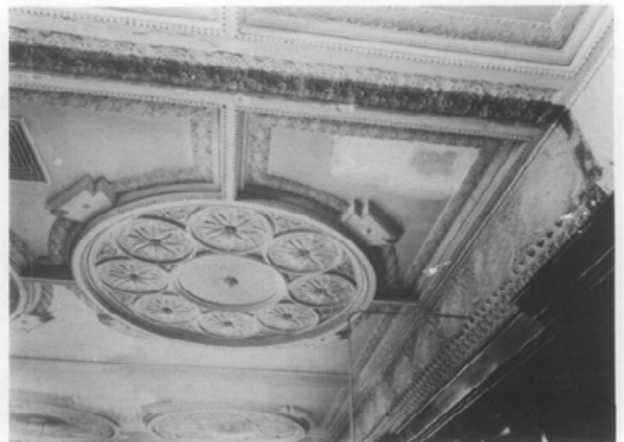
Fig. 16. The Auditorium Building, Chicago, Illinois, 1889, by Louis Sullivan. Earlier insensitive alterations were removed prior to restoration of the room. In the photo, a partition wall has already been removed; the electrical conduit and a ventilation grille followed. Plaster patching and painting were the final steps of restoration work. Photo: National Park Service files.
