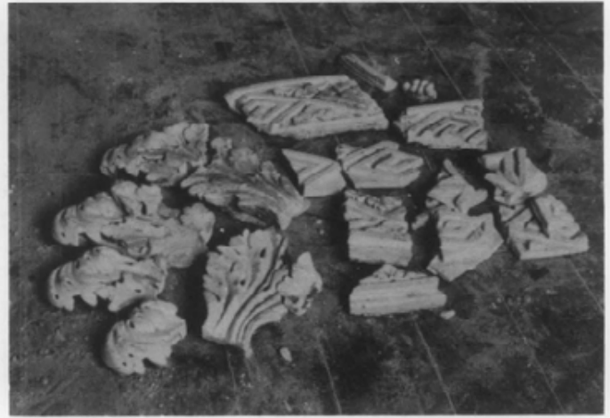
Fig. 19. Ceiling medallions may need repair or replacement. The ornamental plasterer takes impressions of the existing plaster, then casts new plaster elements. Adhesive plaster is used to reattach the new pieces. Left: Damaged elliptical medallion from Rockland, Fairmount Park, Philadelphia, Pennsylvania. Photo: David Flaharty. Right: Fragments of a medallion from the Bennett House, Charleston, South Carolina. The fragments serve as documentation for the replacement medallion. Photo: Peter Sanders.
