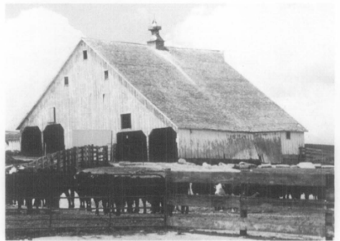
The long, sweeping roof is a characteristic of the Prairie or Western barn. The projecting peak over the hayloft is another. This Iowa barn was built about 1910. Photo: Mary Humstone.
