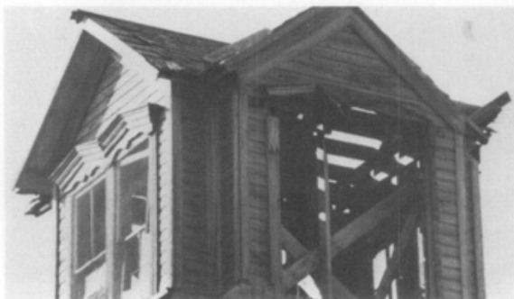
Fig. 8. Built in the Gothic Revival style in the 1890s, this four-story Indiana barn had fallen into disuse, and was deteriorating. In the process of returning it to use, the owner installed a new roof that matches the wooden shingles found beneath the deteriorating asphalt shingle roof; removed the modern asbestos shingle siding; repaired the windows, and reconstructed the cupola (including its lightning rod and weathervane). (Before and after views are of opposite sides of barn.) Photos: Before, Courtesy, Gary Post-Tribune; After, Courtesy, Kankakee Valley News.
