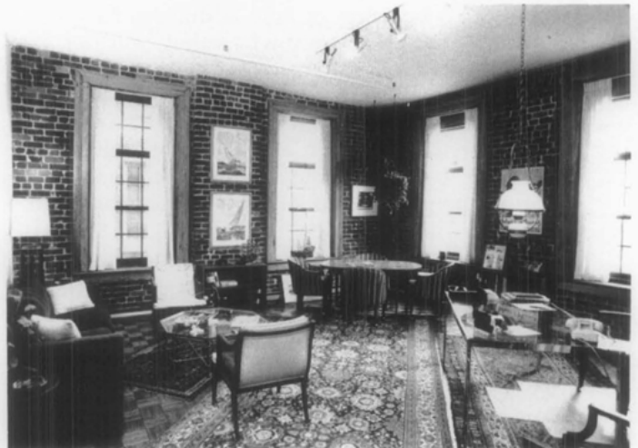
Figure 10. In this case plaster has been removed from perimeter walls, leaving brick exposed. In removing finishes from historic masonry walls, not only is there a loss of historic finish, but raw, unfinished walls are exposed, giving the interior an appearance it never had. Here, the exposed brick is of poor quality and the mortar joints are wide and badly struck. Plaster should have been retained and repaired, as necessary.
