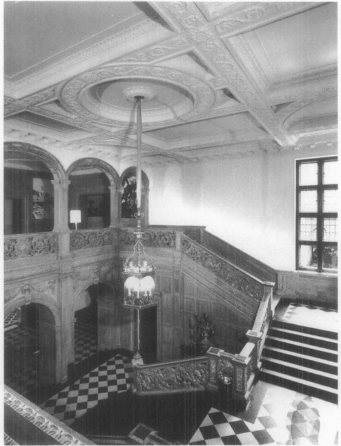
Figure 1. This architect-designed interior reflects early 20th century American taste: the checkerboard tile floor, wood wainscot, coffered ceiling, and open staircase are richly detailed and crafted by hand. Not only are the individual architectural features worthy of preservation, but the planned sequence of spaces—entry hall, stairs, stair landings, and loggia—imparts a grandeur that is characteristic of high style residences of this period. This interior is of Greystone, Los Angeles, California. Photography for HABS by Jack E. Boucher
