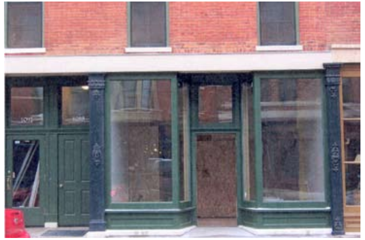
The buildings with compatible new storefronts after rehabilitation with detail of new storefronts.
