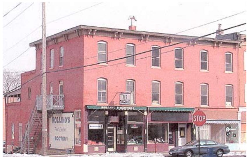
The three buildings prior to rehabilitation.
