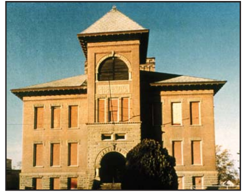
1901 school building prior to rehabilitation.
