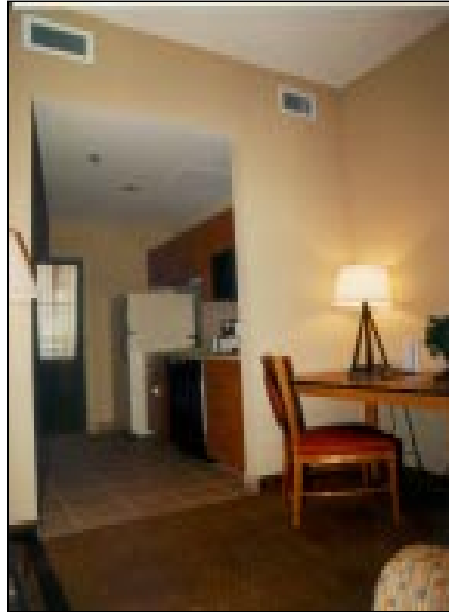
The lowered ceiling in the kitchen area conceals mechanical and other equipment in this rehabilitated 1927 office building.
