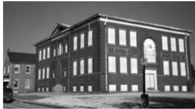
William Shelly School (right) and Annex (left) before rehabilitation. All the original windows remained beneath the plywood.
