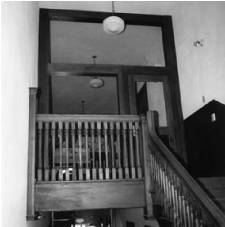
The glass smoke barrier at the top of the stairs is compatible and retains the visual connection between the stairs and the second floor corridor.
