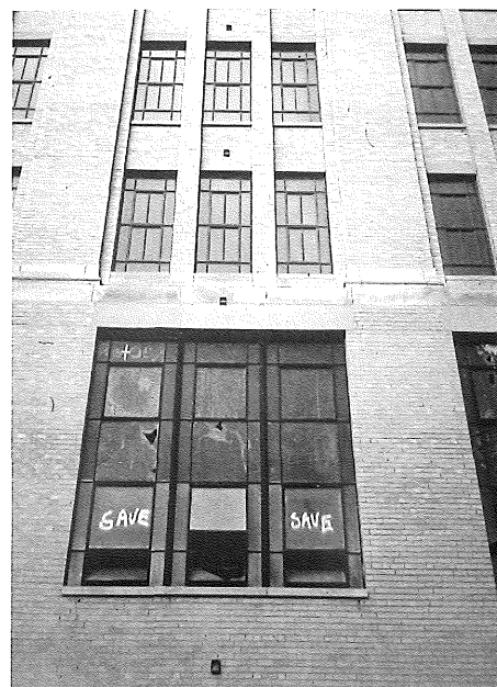
Figure 4. Among the retained and repaired original windows were these large units on the second floor level. Photo: Bruner/Cott & Assoc., Inc.
