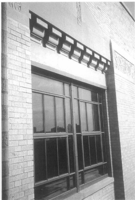
Figure 7. Installed replacement window. Photo: Bruner/Cott & Assoc., Inc.
