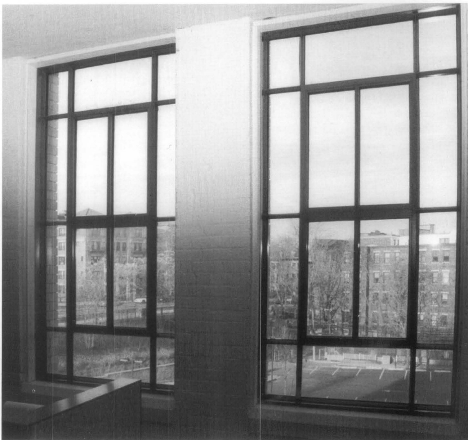
Figure 9. The interior profiles of the original windows were accurately reproduced in the aluminum replacement units. Photo: Bruner/Cott & Assoc., Inc.
