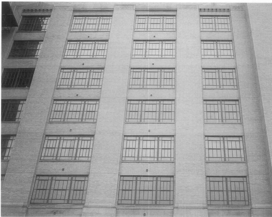
Figure 10. The replacement windows designed for the Sears building rehabilitation met energy efficiency and aesthetic goals while providing for the continued historic appearance of the structure. Photo: Bruner/Cott & Assoc., Inc.
