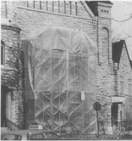
Figure 3. A vinyl cocoon placed over the windows allowed the repair work to be carried out even in inclement weather.
