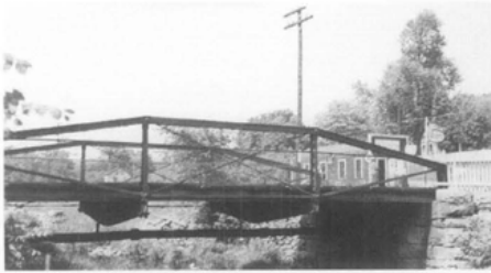
Figure 1. The Stillwater Road Bridge is shown on its original site in Smithfield, Rhode Island, in 1942. Following the decision to replace the historic iron bridge, it was subsequently dismantled, rehabilitated, moved, and re-assembled in nearby Cumberland. Photo: Rhode Island Department of Public Works.
