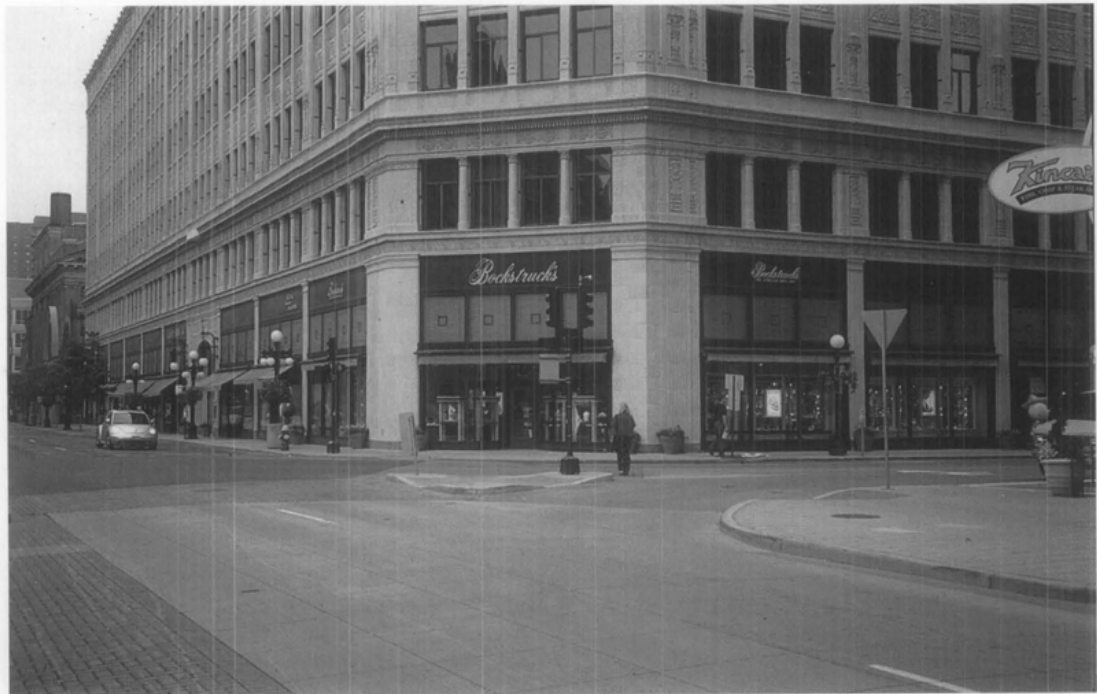
Figure 2. The Hamm Building featured fifty-six prismatic panels set directly above the awnings. Each panel contained over two hundred individual tiles. Photo shows completed project. Photo: Chad Randl
