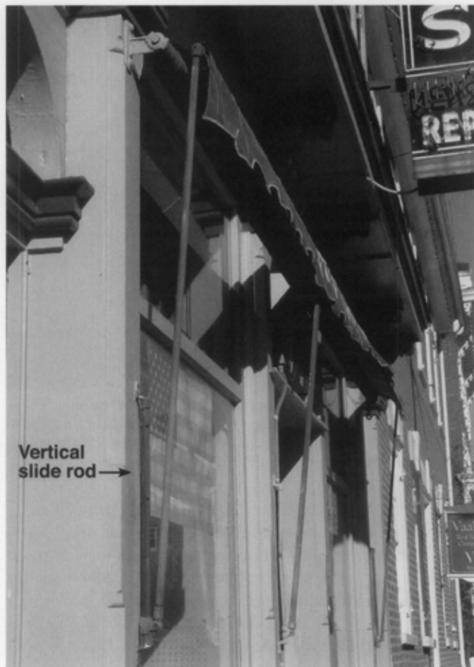
Figure 8. The roller bar at the top of a fixed-arm awning is cranked to release the fabric. As the canvas unfurls the vertical arms swing downward from their lower point. Because the pictured awning had a large projection, extending far from the building wall, the lower hinges were mounted on vertical slide rods affixed to the facade. When the awning is lowered, the bottom hinges of the arms travel up the slide rod to increase headroom beneath the fully extended awning.
