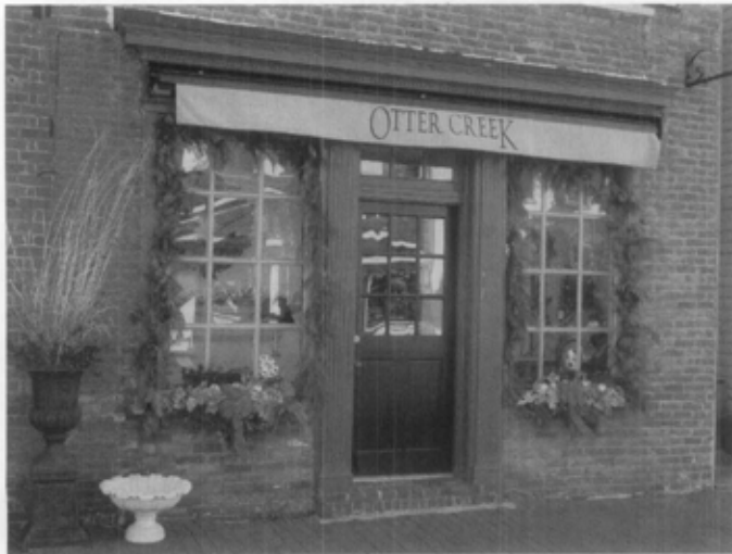
Figure 25. Appropriate lettering, as on this roller awning valance, can function as distinctive signage without detracting from the historic character of the building.
