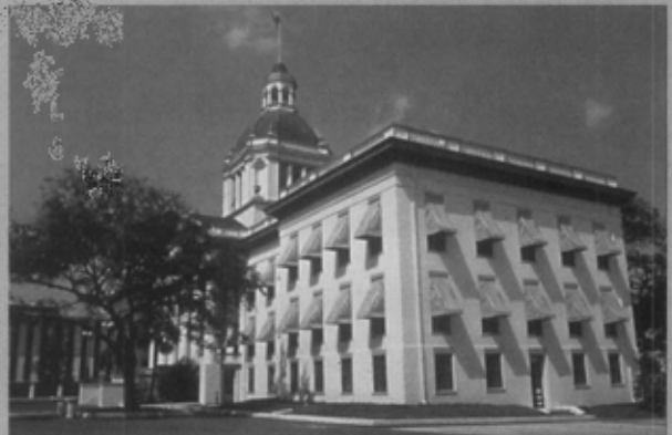
Awnings were reinstalled on the east, west, and south windows of the Florida State Capitol in the 1980s. With a design based on those seen in historic photographs of the building, the new awnings allowed a downsizing of the HVAC system by 25 tons. After installation, the exposed glass surface in a typical first floor office accounted for only 46% of the required cooling load, down from 72%. Photo: Division of Historical Resources, Florida Department of State.
