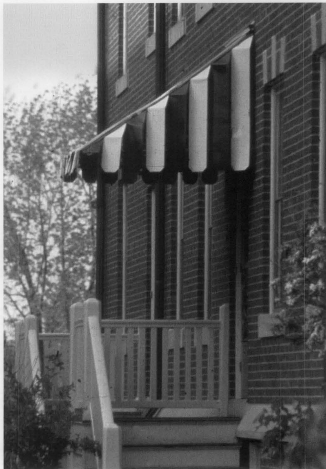
Figure 23. This postwar aluminum awning does not contribute to the character of this 19th century residence and could be replaced during a rehabilitation project with a fabric shed awning more in keeping with the building's age and appearance.
