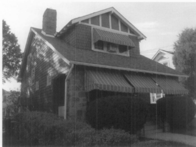
Figure 19. Simple shed-type awnings with acrylic or canvas coverings and free-hanging valances are appropriate for most historic residences featuring rectilinear openings.
