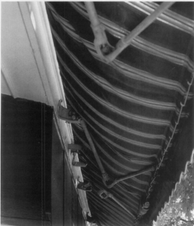
Figure 13. Lateral-arm awnings were preferred on long elevations, especially those with sheet glass (where vertical arms could not be fastened to the building facade). When lateral arm awnings were installed across a broad storefront or porch, manufacturers recommended spacing the arms at approximately eight foot intervals.
