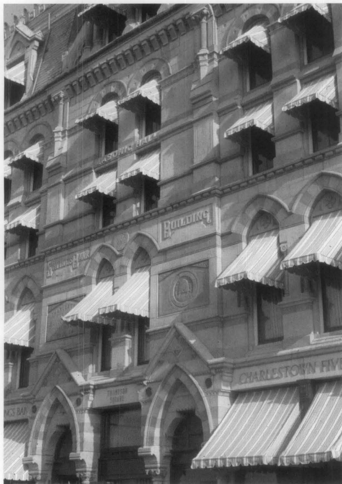
Figure 22. These window awnings today match what would have appeared in the 19th century. The fabric is slightly loose on the frames, the valances hang freely, each window bay has its own awning, and the awning frames are set within the openings. Photo: Mike Jackson.
