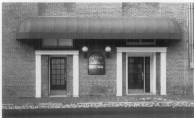
Figure 21. Single awnings should not be set over more than one door or window bay. A separate shed awning with a canvas or acrylic covering would be more appropriate over each of these openings.
