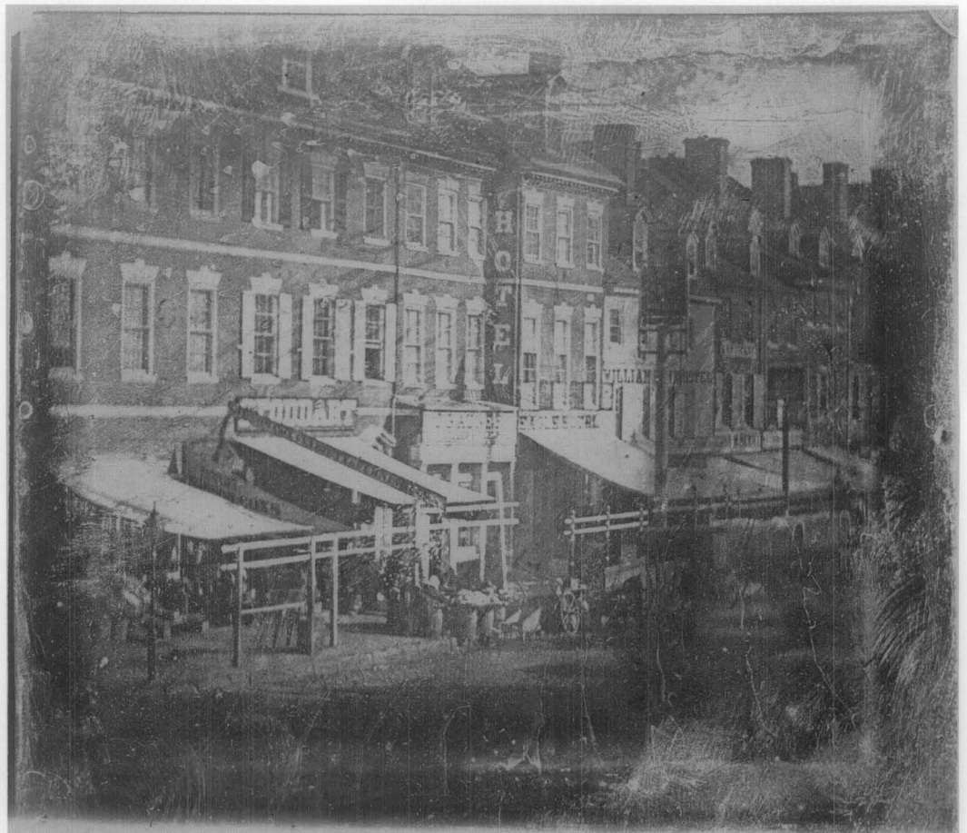
Figure 3. Early 19th century awnings featured canvas coverings stretched between the building facade and post-supported front bars. Projecting frameworks of extension bars were not common until later in the century. Photo: Second Street, Philadelphia, c. 1841, Print and Photo Collection, The Free Library of Philadelphia.
