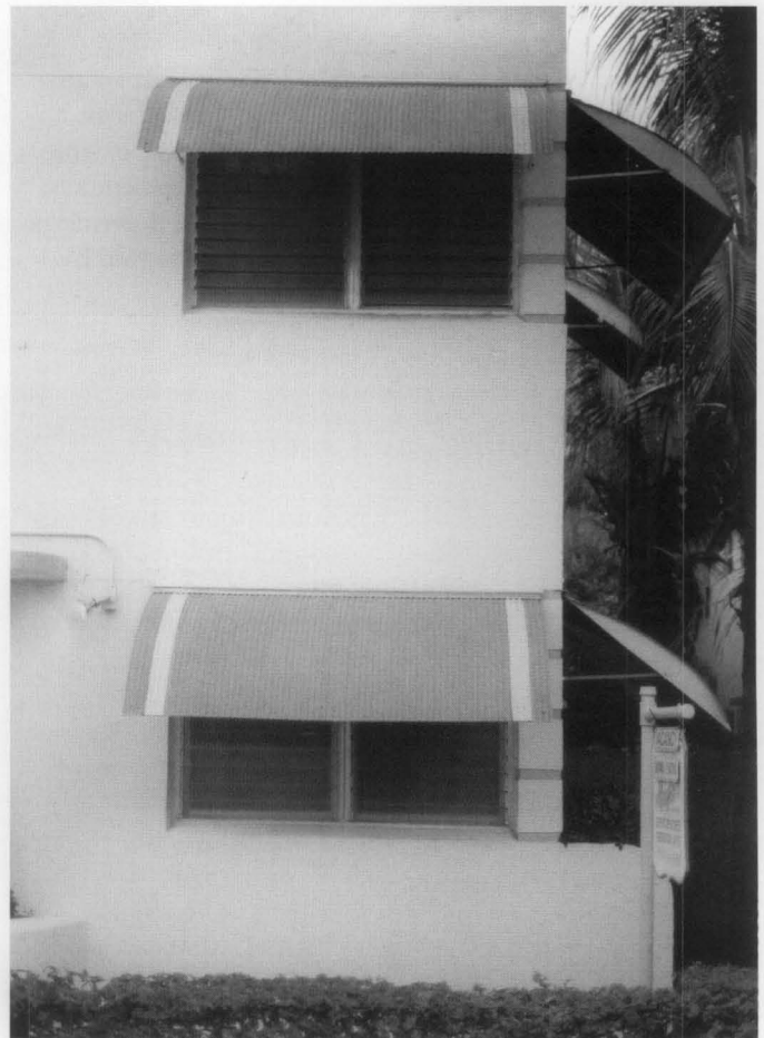
Figure 16. These fiberglass "clamshell" awnings, although not as old as the 1930s building to which they were affixed, are important features that have acquired significance. They were retained when the building was recently rehabilitated.
