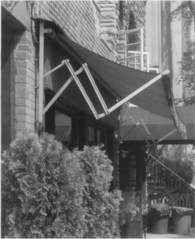
Figure 12. Scissors-arm awnings have a pair of vertical, hinged arms on either side of the assembly supporting the front bar. To unfurl the awning, the roller is cranked and the arms extend outward pulling the cover away from the roller.
