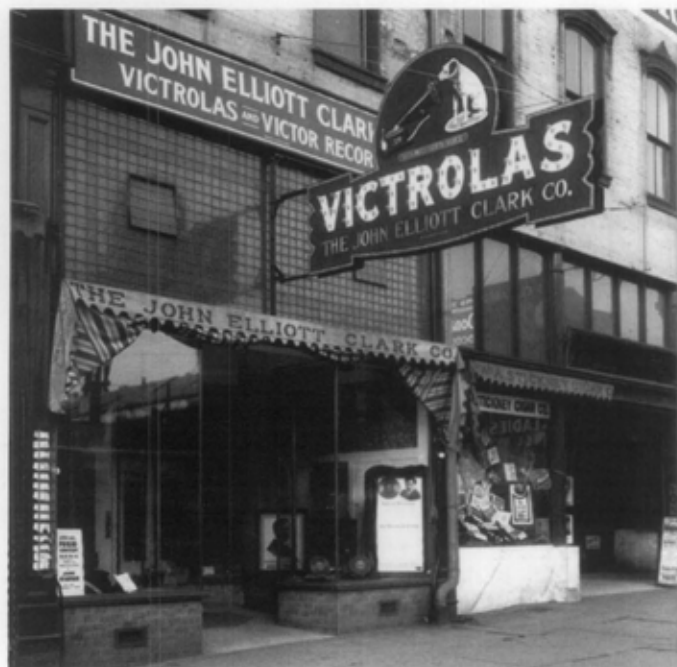
Figure 7. Early 20th century photo showing two operable awnings, an early version on the left and a next-generation roller awning on the right. The roller awning, with no side panels and just the valance showing, presented a clean storefront appearance. Photo: Utah State Historical Society, used by permission, all rights reserved.
