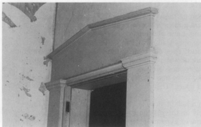
Fig. 5 (a). The photo above shows the use of wooden plaster "grounds" nailed to the wall studs of the mid-19th century Lockwood House in Harpers Ferry, West Virginia. This allowed the plasterer to work flush with the surface of the grounds. Afterwards, the carpenter could nail the finish woodwork to the ground, effectively hiding the joint between the plaster and the ground. The trim was painted after its installation, leaving a paint outline on the plaster. Fig. 5 (b). The photo below shows door trim and mouldings in place after the plastering was complete. Photos: Kay Ellen Simonson.
