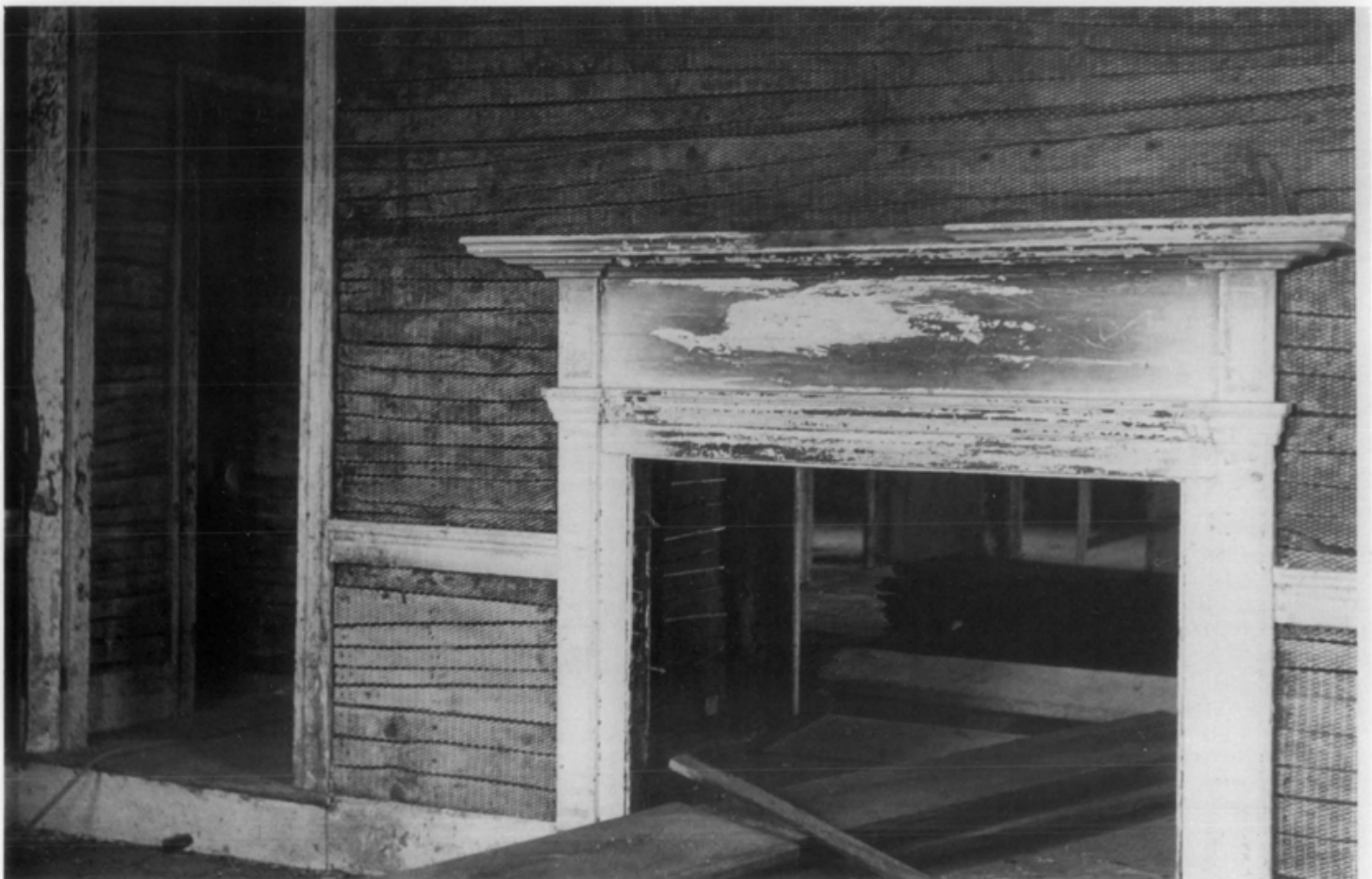
Fig. 16. In the restoration of a ca. 1830s house in Maine, split-board lath has been covered with expanded metal lath in preparation for new coats of plaster. This method permits the early lath to be saved while the metal lath, with its superior keying, serves as reinforcement. Photo: National Park Service files.
