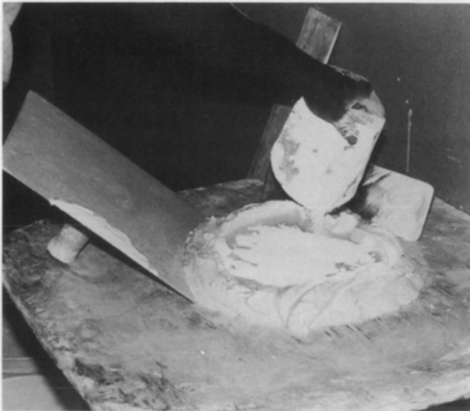
Fig. 17. This contemporary plasterer is mixing a lime finish coat in much the same way as America's earlier artisans. The ring consists of lime putty; the white powder inside is gauging plaster. After the mixture is blended, a steel trowel will be used to apply it. It should be noted that a traditional lime finish coat can be applied over a veneer plaster base coat to approximate the look of historic plaster walls and ceilings. Photo: Marylee MacDonald.
