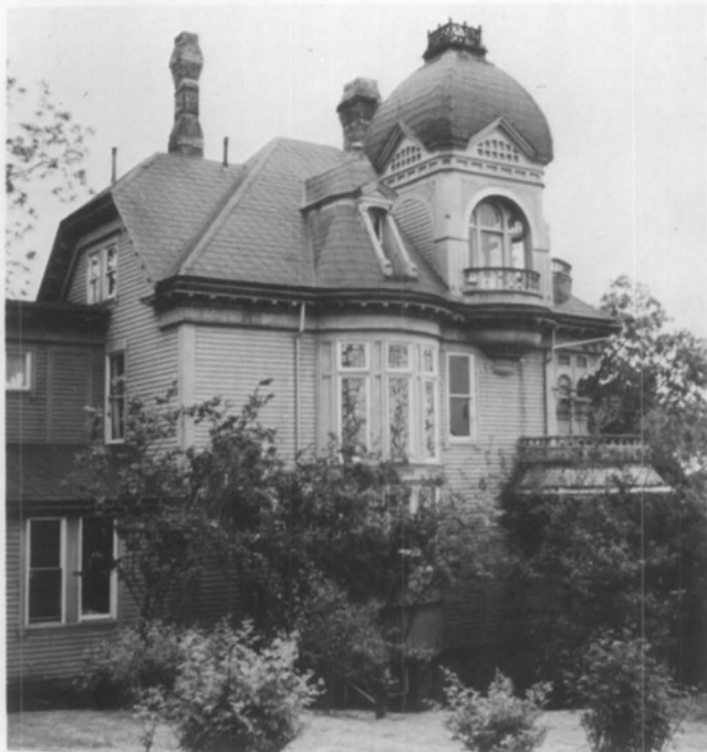
Special problems inherent in the design of an elaborate historic roof can be controlled through the use of good materials and regular maintenance. The shape and detailing are essential elements of the building's historic character, and should not be modified, despite the use of alternative surface materials. (Gamwell House, Bellingham, Washington)
