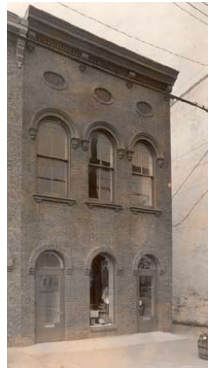
The storefront on this Victorian building prior to rehabilitation was a later replacement (left). During rehabilitation the storefront was removed and replaced with three residential-type openings that are incompatible with the building's retail character (right).
