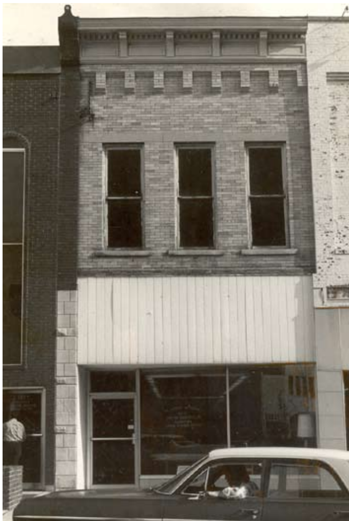
Prior to rehabilitation this early-20th century commercial building had a 1950s storefront (left). Rehabilitation plans proposed replacing the storefront with 18th century-style residential-type openings, inappropriate for this commercial building and its period of construction (right).
