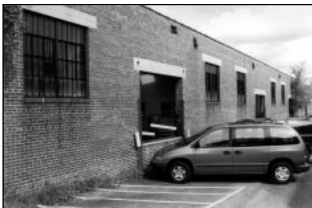
Loading door elevation after rehabilitation.
