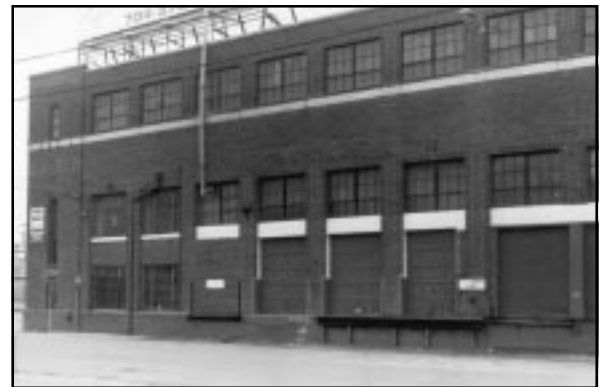
Cargo bay doors are incorporated within the fenestration rhythm. Some of the existing openings have been enlarged and later metal roll-up doors installed.
