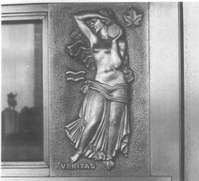
Figure 49. Monel and Nickel Silver Doors, United Nations General Assembly Building, First Avenue between East 42nd and 48th Streets, New York City, 1953; Ernest Cormier, designer, Montreal. The contrasting pale yellow nickel silver and platinum-colored Monel metal doors were a gift from Canada to the United Nations. The seven nickel silver doors were fabricated from extruded sections by the Anaconda American Brass, Ltd.; and the Monel metal sculptural panels representing Truth, Peace, Justice, and Fraternity were cast by Robert Mitchell Company, Ltd. (David W. Look)
