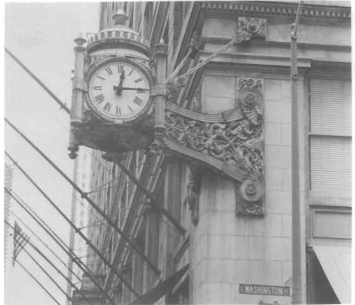
Figure 29. Bronze Clock, Marshall Field and Company Department Store Addition, corner of State and East Washington Streets, Chicago, Illinois, 1907; Graham, Anderson, Probst & White, architects. This huge bronze clock, weighing 7 3/4 tons and hanging 17 feet above the sidewalk, was designed by Pierce Anderson for the addition to Marshall Field's store. With a 46-inch face and a minute hand measuring 27 inches, the clock and its twin on another corner of the building can be seen for blocks. These magnificent works of art have become part of the city's landscape as a fourth generation of Chicagoans meet "under the clock." (Margot Gayle)
