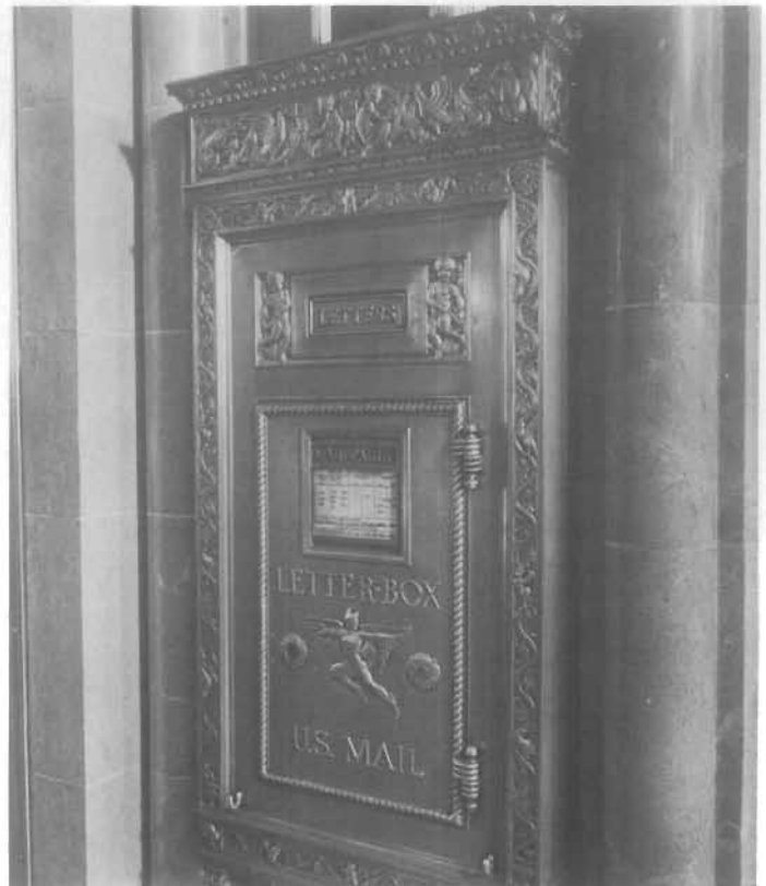
Figure 30. Bronze Teller Cage and Mailbox, Bowery Savings Bank, 110 East 42nd Street, New York City; 1923, York and Sawyer, architects; William H. Jackson Co., foundry. The Bowery Savings Bank has been relatively unscathed by "modernizing" and is literally filled with bronzework: doors, elevators, check writing desks, window trim, tellers' cages, gates, and even mailboxes. (a) Although the function of tellers' cages was to provide security, they were transformed into decorative features. (b) During the late 19th and early 20th centuries, functional items such as letter boxes were custom designed for each building and integrated into the total design. (Bowery Savings Bank)
