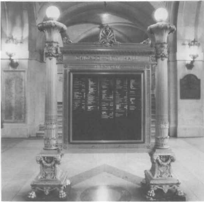
Figure 38. Brass Lobby Directory, City Hall and County Building, Chicago, Illinois, 1911; Holabird and Roche, architects. A dual purpose lobby directory and light standard, this piece of brass lobby "furniture" displays the capacity of brass to take the most opulent and ornamental cast shapes. This design is in keeping with the elaborate style of many neoclassical buildings erected in the early years of this century. (Office of the Mayor, City of Chicago)
