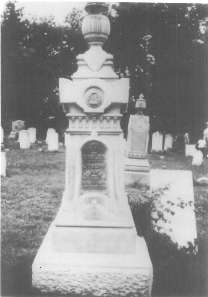
Figure 14. Zinc Grave Marker, Herkimer, New York, ca.1874; Monumental Bronze Co., Bridgeport, Connecticut. The manufacturer's name is discreetly recorded in small letters along the edge of the plinth. This company's 1882 catalog used the phrase "pure cast zinc" while insisting that "unlike commercial zinc ours is a pure metal, like gold or silver." The embossed epitaph is still crisp and new looking. In some respects the zinc monuments have survived in better condition than their stone counterparts. These light gray markers were cast in many sections, sandblasted to produce a rough stone-like surface, then bolted together with the connections disguised. (Margot Gayle)
