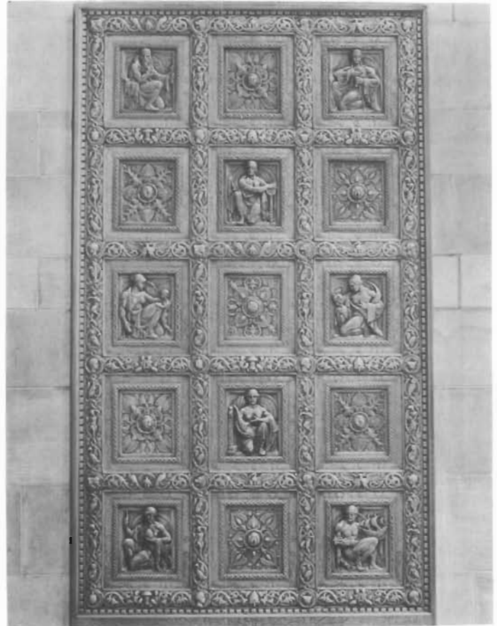
Figure 2. Bronze Entrance Door, Bowery Savings Bank, 110 East 42nd Street, New York City, 1923; York and Sawyer, architects; William H. Jackson, foundry. Cast in the boom era after World War I, this main entrance door reflects the aura of success and stability bank officials sought. The color of polished bronze probably accounts for its use as much as its permanence and molding qualities. This is a good example of a building in which art, architecture, and sculpture were combined in an overall concept down to the smallest detail. (Courtesy of the Bowery Savings Bank)
