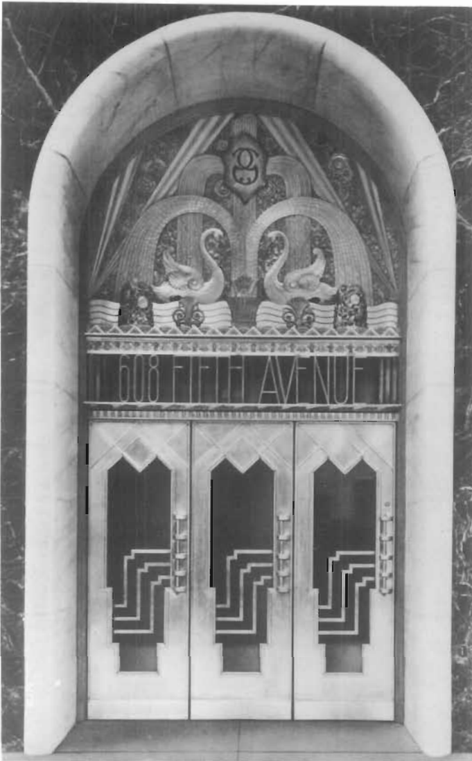
a. Figure 46. Nickel Silver Doors and Tympanum, Golet Building, New York City, 1932; E. H. Faile, architect; General Bronze Corp., foundry, Long Island, New York. (a) This Art Deco-style entrance features silvery-yellow geometric doors which are almost overshadowed by the exuberant swan and fountain design in the tympanum with its array of colorful shapes. (b) The effect was achieved with a combination of copper, bronze, brass, nickel silver, and black enamel as indicated on the original drawing. When the first-floor facade was remodeled in 1966, the doors were removed and stored; the tympanum was taken to Newport, Rhode Island, to be reinstalled in a private club. (International Nickel Company)
