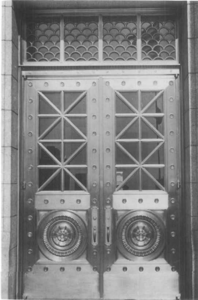
Figure 40. Brass Doors, Utah State Capitol, Salt Lake City, 1913-1916; Richard Kletting, architect. Brass was not used for exterior doors as often as bronze, although many doors that are reportedly bronze may actually be brass. These highly polished exterior brass doors, make a strong architectural statement reinforcing the overall design of the building. Classical motifs include Roman grate windows, circular shields in the lower panels, and a scallop design in the transom. (Margot Gayle)
