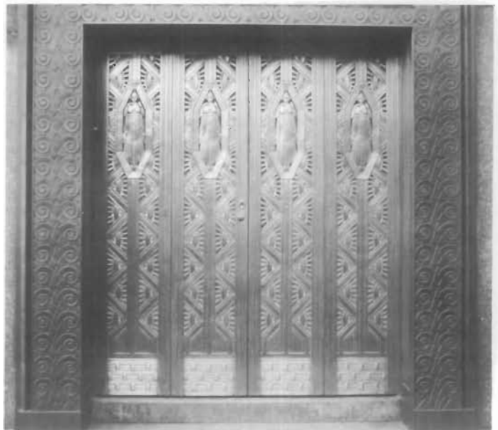
Figure 42. Nickel Silver Doors, Manufacturers Hanover Trust, 481 Seventh Avenue, New York City, 1930; Sugarman and Berger, architects. Cast in yellow nickel silver, the Art Deco style doors on this bank look like brass and are in striking contrast to the bronze door surround and red granite walls. (David W. Look)
