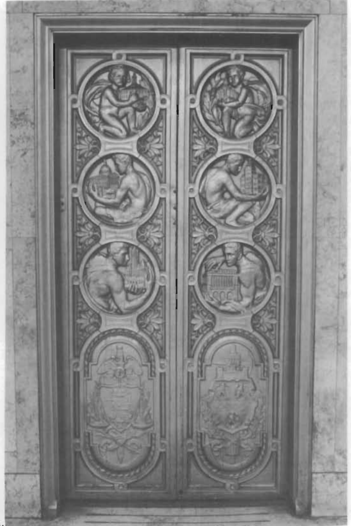
Figure 39. Brass Elevator Doors and Brass-Sheathed Columns, City-County Building, Pittsburgh, Pennsylvania, 1915-1917; Palmer, Hornbostel and Jones, architects; Edward B. Lee, associate architect; Tiffany and Co., designers (for columns only). (a) Brass was used extensively for interior decorative features in 19th- and 20th-century buildings, and was especially popular for statuary, large-scale furniture, and elevator doors in government and office buildings. This set of highly modelled brass doors tells the story of Pittsburgh's development as reflected in its important buildings. (b) The large structural steel columns that support the barrel vault of the lobby are sheathed in brass—an unusual choice of material for columns. Over the years the fluted shafts and stylized capitals had acquired a dull, dark patina, but when the lobby was restored in 1972, the columns were polished and lacquered to return them to their original appearance. (Pittsburgh History and Landmarks Foundation)
