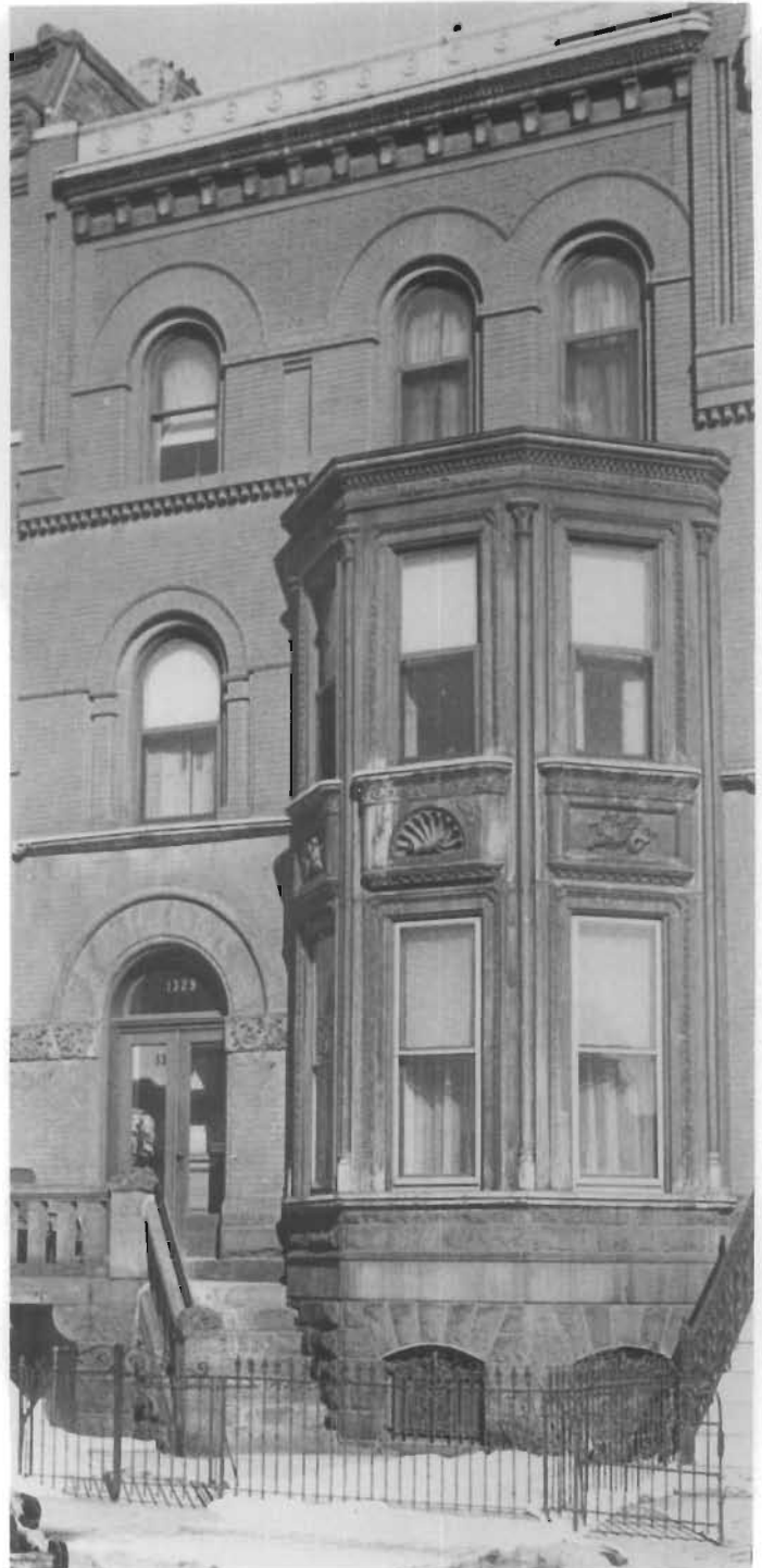
Figure 24. Copper-Clad Bay Window and Cornice, Thomas C. Whyte House, 1329 R Street, NW, Washington, D.C., 1892; George C. Johnson, architect. From the first-floor window sills to the cornice above the second floor, the bay window is sheathed entirely with pressed sheets of copper, and there are slender two-story copper pilasters flanking the windows. The spandrel between the first- and second-floor center windows has a shell design and the side spandrels have winged sea creatures. Both the cornice of the house and the cornice of the bay window have copper classical dentils and modillions. (David W. Look)
