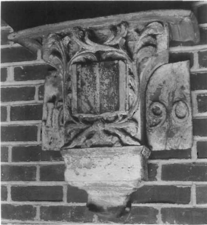
Figure 5. Lead Rain Conductor Head, Library Hall, Philadelphia, Pennsylvania, 1789–1790; from designs of Dr. William Thornton. When the library was razed in 1884, this conductor head was saved and became part of the collection of the Library Company of Philadelphia. Many early rain conductor heads were constructed of lead, and frequently included date flanges, as seen here. However, this is the only known example of a lead conductor head with an “open book” motif. (Jack E. Boucher)
