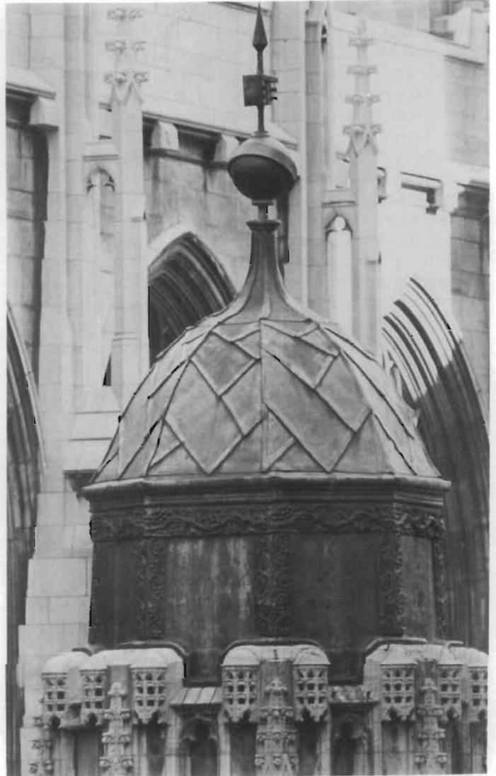
Figure 6. Lead Roofing, Saint Thomas Church, Fifth Avenue and 53rd Street, New York City, 1909–1914; Cram, Goodhue, and Ferguson, architects; Henry Hope and Sons, lead craftsman. Ralph Adams Cram designed St. Thomas Church using the spirit and many of the techniques of medieval builders, including the use of small overlapping sheets of lead for roofing curved surfaces. The decorative grapevine frieze and panel borders, also of lead, show the versatility of this material, which can be cast with sharp detail. (Becket Logan)
