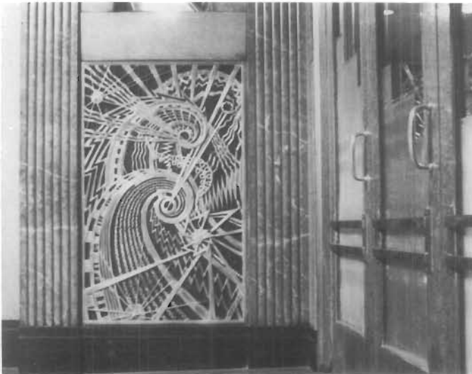
Figure 33. Bronze Ventilation Grille, Chanin Building, 405 Lexington Avenue, New York City, 1929; Sloan and Robertson, architects; lobby design by Jacques Delamarre. The foyer of this Art Deco style building contains four highly modeled ventilation grilles in an abstract design, in what some designers called the "Futuristic" style. (David W. Look)
