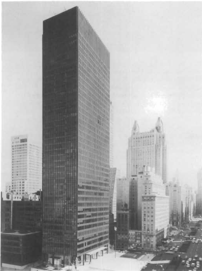
Figure 34. “Bronze” Curtain Wall, Seagram Building, 375 Park Avenue, New York City, 1958; Ludwig Mies Van der Rohe, architect. The curtain wall consists of 4 1/2- by 6-inch extruded architectural “bronze” (really brass: 57% copper, 3% lead, and 40% zinc) I-beam mullions (2 1/2 inches larger than the largest bronze sections extruded to that time), Muntz metal spandrels (brass also: 60% copper and 40% zinc), and pink-gray, heat- and glare-resistant glass in story-high architectural bronze frames. The 26-foot-long architectural bronze I-beams were extruded rather than built up with welded plates to avoid waviness in the sections. The architectural bronze, which only resembles real bronze with a statuary brown patina in color, is regularly rubbed with oil to prevent the bronze from forming a natural green patina. (Ezra Stoller)
