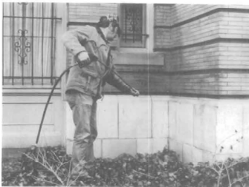
Figure 7. A contractor prepares equipment before testing a low-pressure water wash on a Roman brick and terra cotta building. Photograph: Sharon C. Park, AIA
