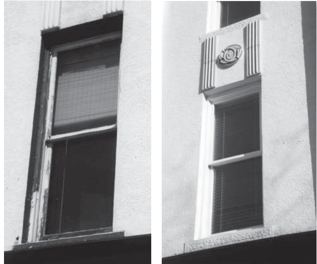
Before/after. Window sash on the street elevations were repaired and retrofitted with a piggyback interior energy panel.
