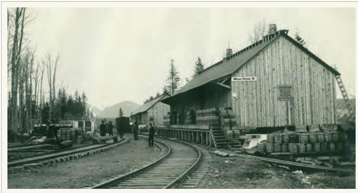
The Alaska Central Railway built a series of warehouses along Seward's waterfront to supply the railroad's construction needs. Photo by Evans: Resurrection Bay Historical Society, Winter Collection, cropped from original.
