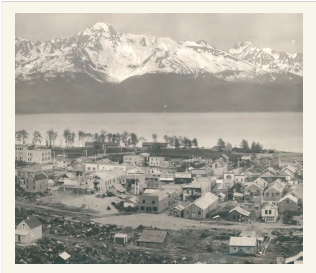
Block 10, circa 1915. The house with the false front at right in photo is the Leslie House. Running from right to left from this house: Harvey cottage, Graef warehouse and Sheal/Graef cottage. Photo by F.W. Sheelor: Seward Community Library Association, cropped from 1915 panorama.
