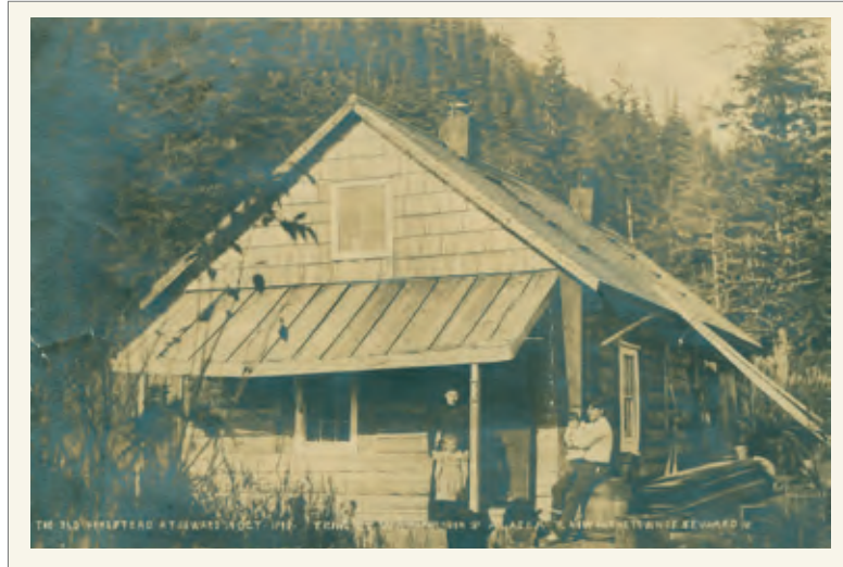
The Lowell family cabin, one of a number of structures on the Lowell homestead at the head of Resurrection Bay. Photo by W.A. McPherson: Resurrection Bay Historical Society, 21.1.4.
