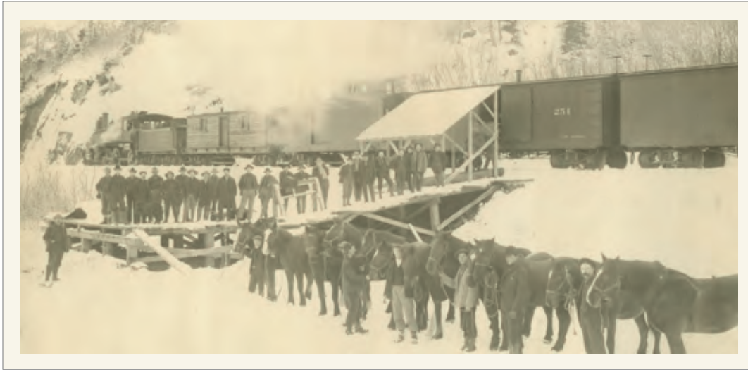
By November 1906 track had been laid to mile 49, just beyond Tunnel No. 1. Here railroad workers arrived from, and departed for, Seward. Photo by Evans: Resurrection Bay Historical Society, Winter Collection, cropped from original.
