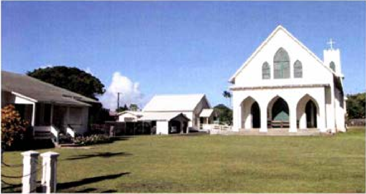
Figure 18. St. Francis Catholic Church complex showing rectory, garage, community hall and chapel.
