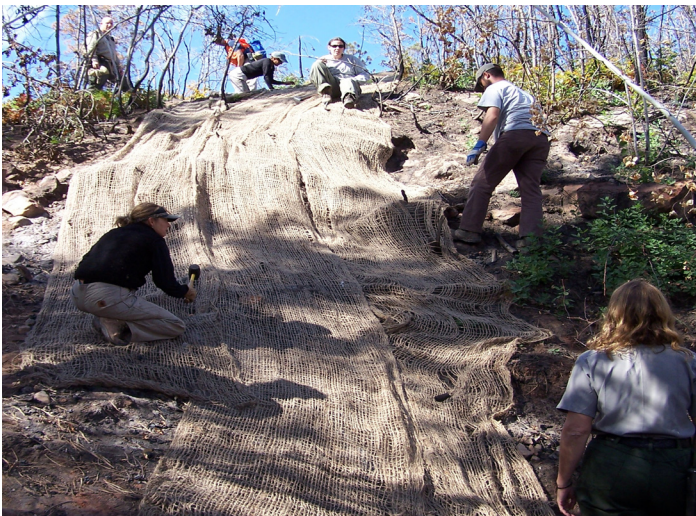
Erosion control rehabilitation
