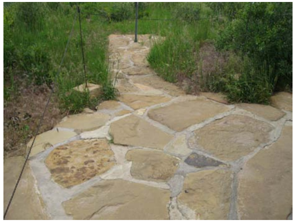
Restored flagstone walkways
