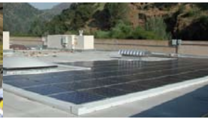
Solar array on the NPS operations complex in El Portal
