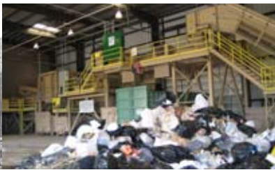
Mariposa County composting facility turns garbage into landfill cover
