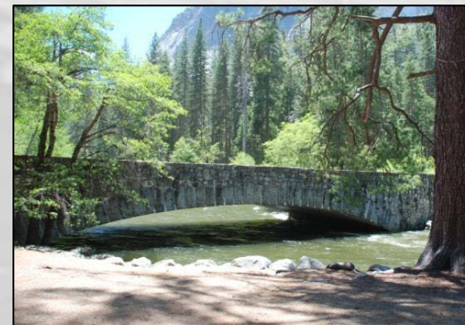
Hydrologic impacts of Sugar Pine Bridge
