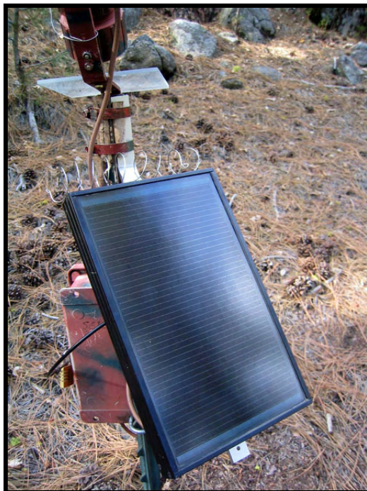
Figure 4. Spring wire helix on solar panel upper margin to lessen bird guano deposition, 19 Sept 2007.
