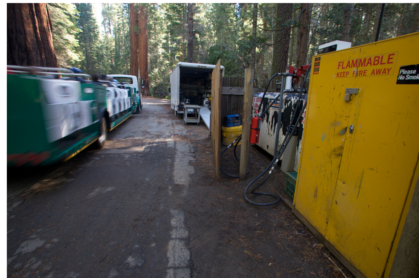
Fuel storage tanks for the tram are located beneath the giant sequoias.
