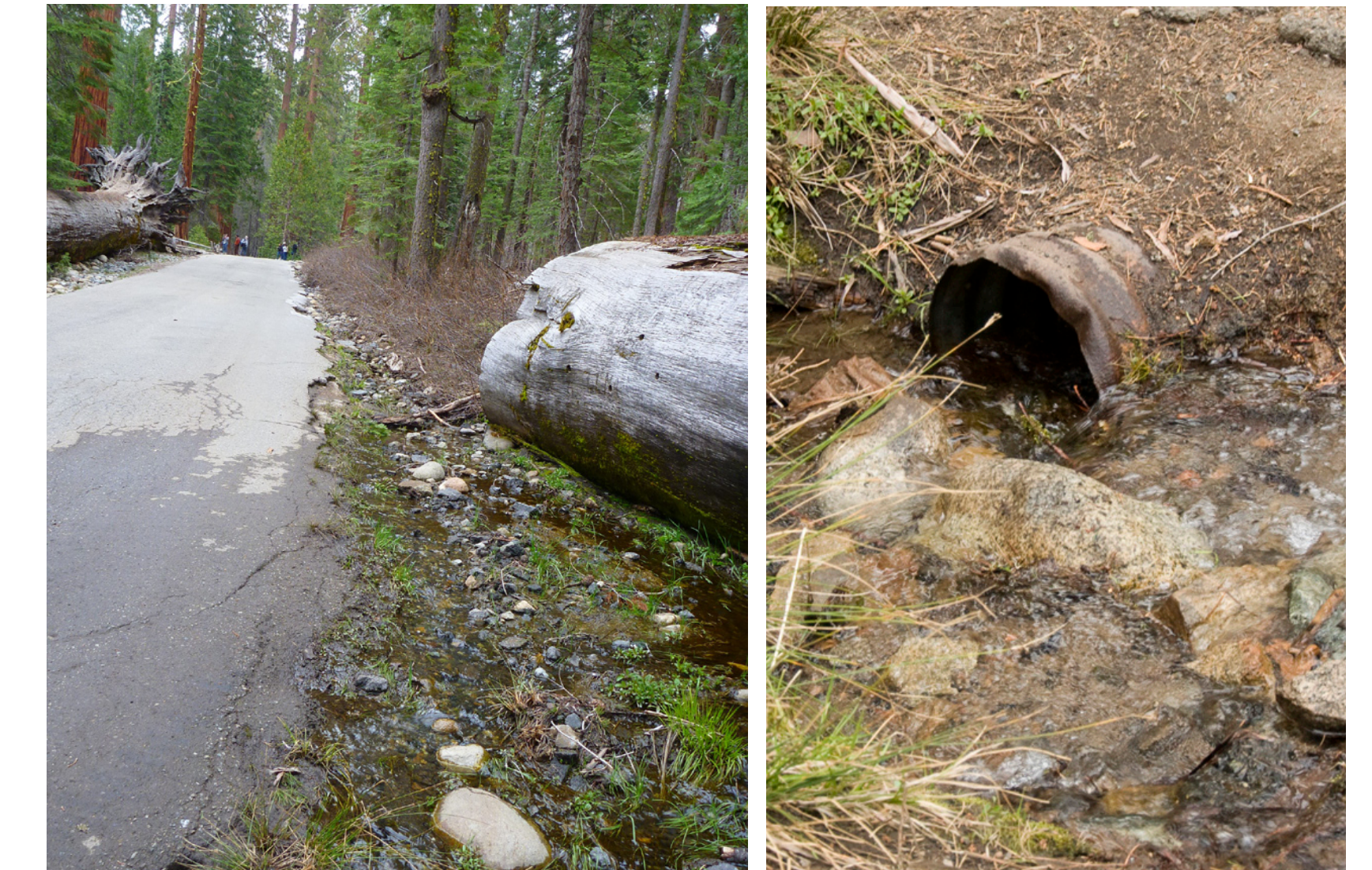
Paved roads throughout the Grove disrupt the surface water needed by the sequoias.
