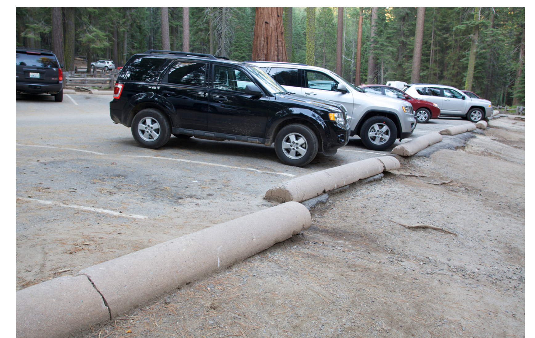
Stormwater runoff from roads and parking areas runs directly into the surrounding forest.
