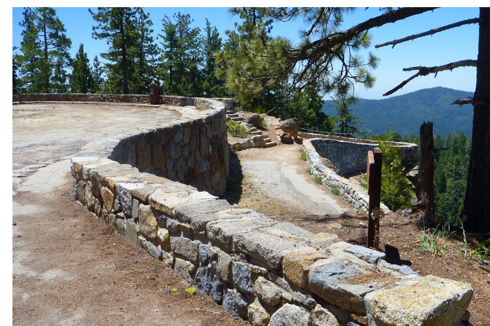
Wawona Point, a significant example of National Park Service landscape architecture of the 1930s, is in a state of disrepair.
