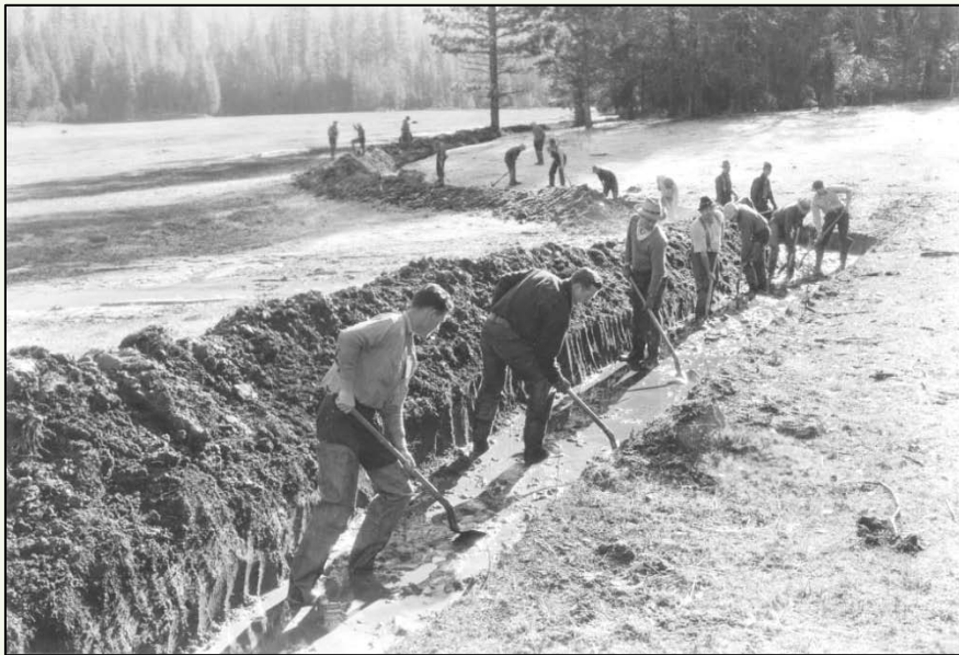
CCC crews clearing drainage ditches in Wawona Meadow
