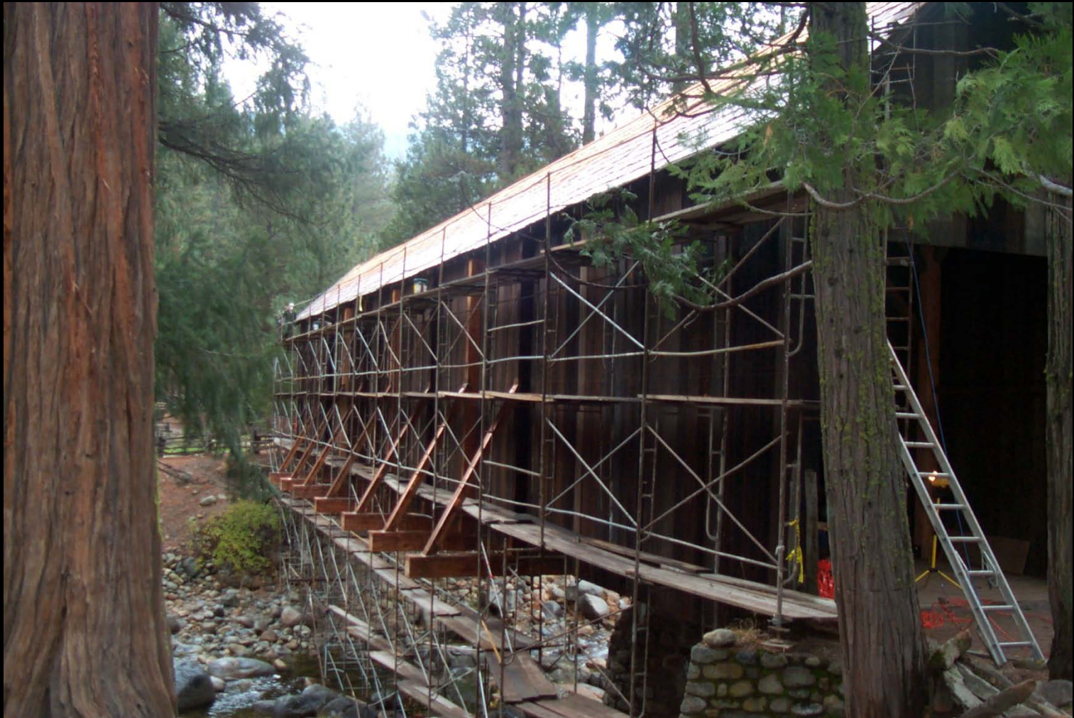
Wawona Covered Bridge 1999 Repair Project
