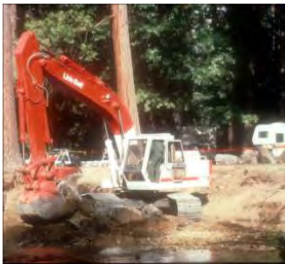
Figure 2: Restoration staff using excavator to remove riprap at Lower River Campground.
