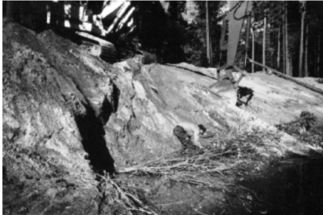
Figure 1: Crew member planting willow and cottonwood cuttings with the aid of the excavator
