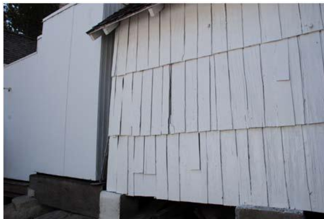
Figure 7. Deteriorating wood-shingle siding
