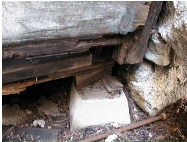
Figure 6. Erosion and settling of foundations
