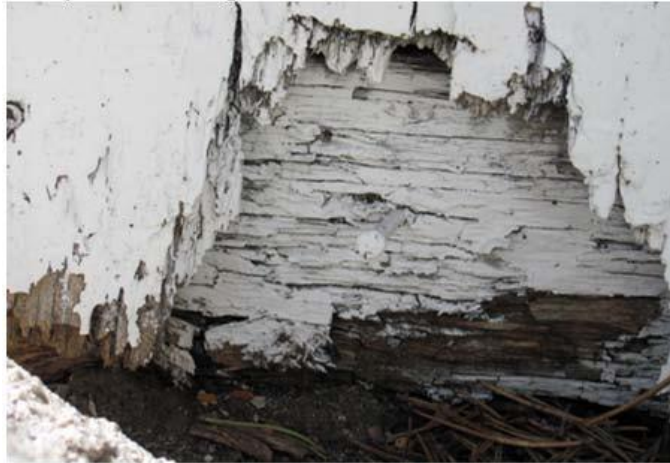
Figure 8. Decayed exterior wall
