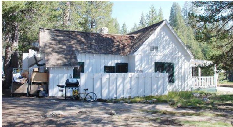
Figure 3. White Wolf Lodge Main Lodge building, south view
