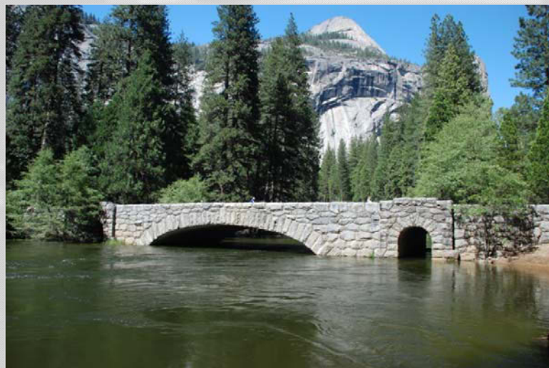
Stoneman Bridge at high water
