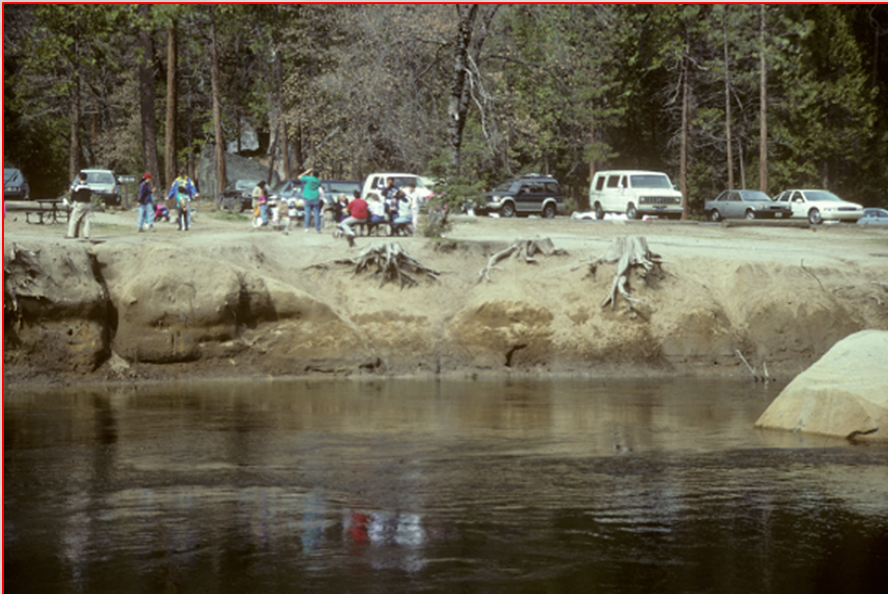
Devil's Elbow, pre-restoration, 1993
