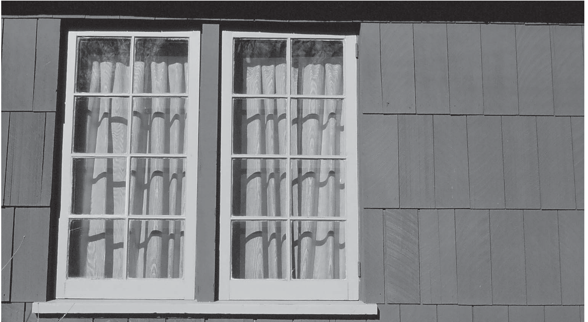
Figure 7.2: Eastern elevation gabled end (Jaramillo, 2009)
