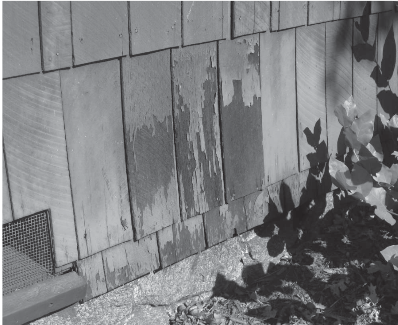
Figure 6.11: Water damaged siding, possibly due to snow accumulation. Note the original brown stain underneath the painted surface. (Summers, 2009)
