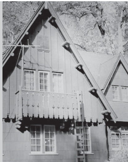
1967 Existing fire escape ladder
