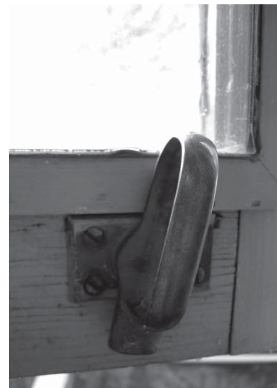
Figure 6.31: Above, original window screen scalloped hinge. Below, Window brass latch (Jaramillo, 2009)
