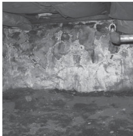
Figure 6.6, clockwise from left: Foundation stone pier footing and post, reinforced foundation, existing stone foundation with efflorescence, note moisture on ground (Summers, 2009)
