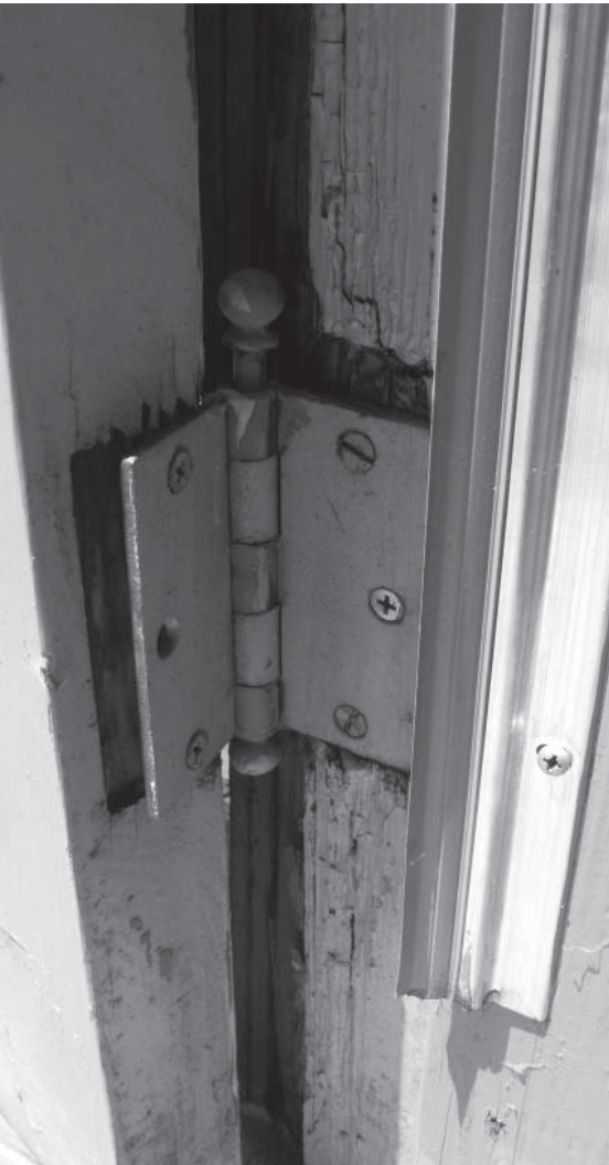
Figure 6.35: Damaged hinged and evidence of moisture on terrace door. Note the added weatherstripping to the door leaf. (Jaramillo, 2009)
