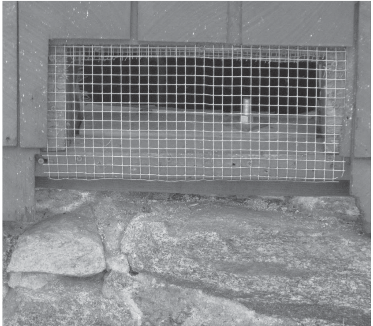
Figure 6.7: Crawlspace vent with added 1/4" metal screen. Although this treatment has kept some pests out it also keeps many of them in. (Jaramillo, 2008)
