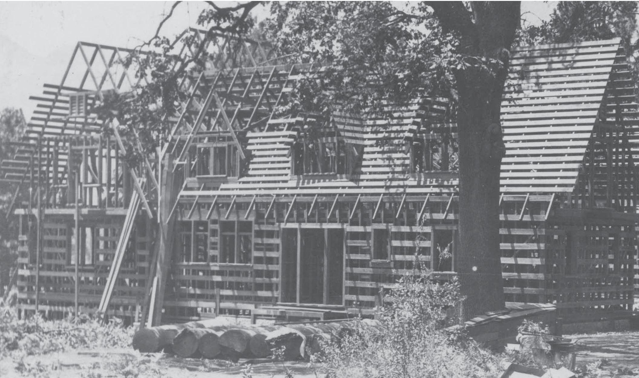
Figure 3.17: Construction of the Rangers' Club, 1919 (YRL 6025)
