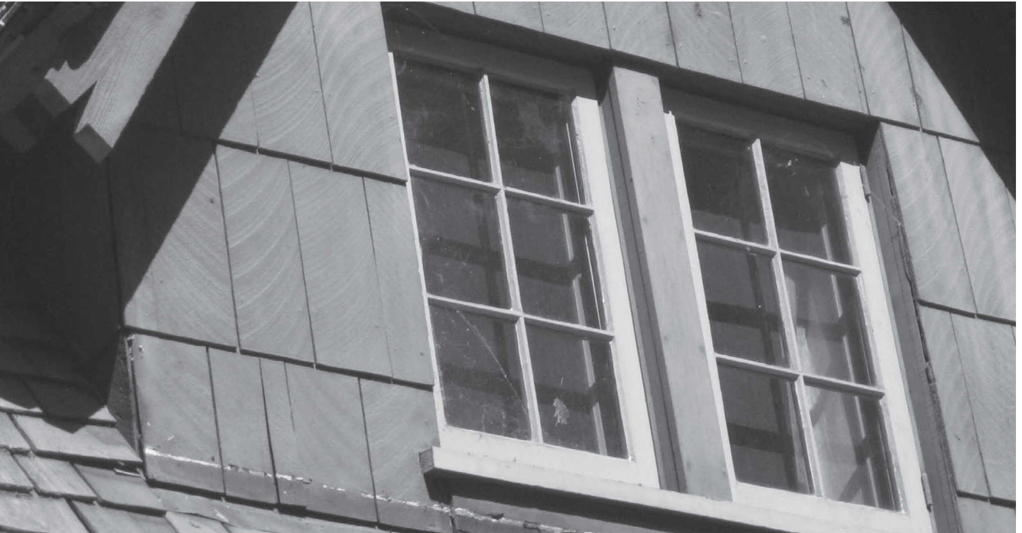
Figure 6.18: Dormer window on west courtyard elevation. Note lower row of shingles with damaged base. (Jaramillo, 2009)
