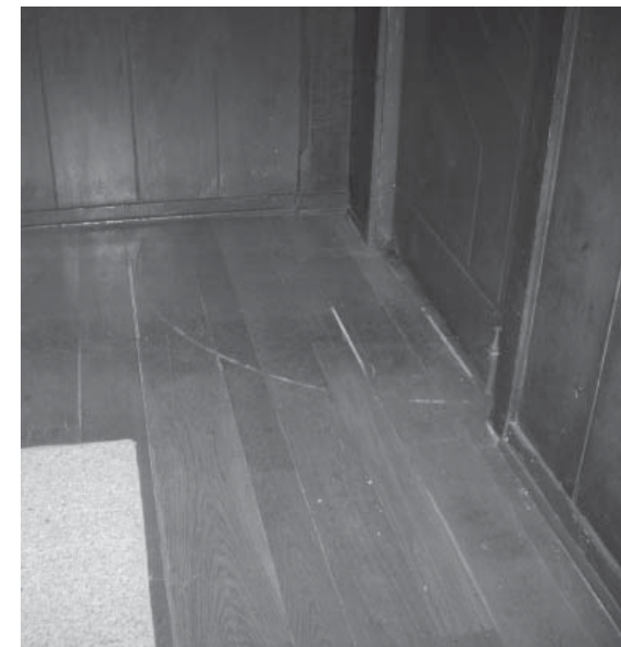
Figure 6.43: Above, Damaged floor at terrace doors, below, damaged and scuffed floor at kitchen entry (Jaramillo,2010, Sommers, 2009)
