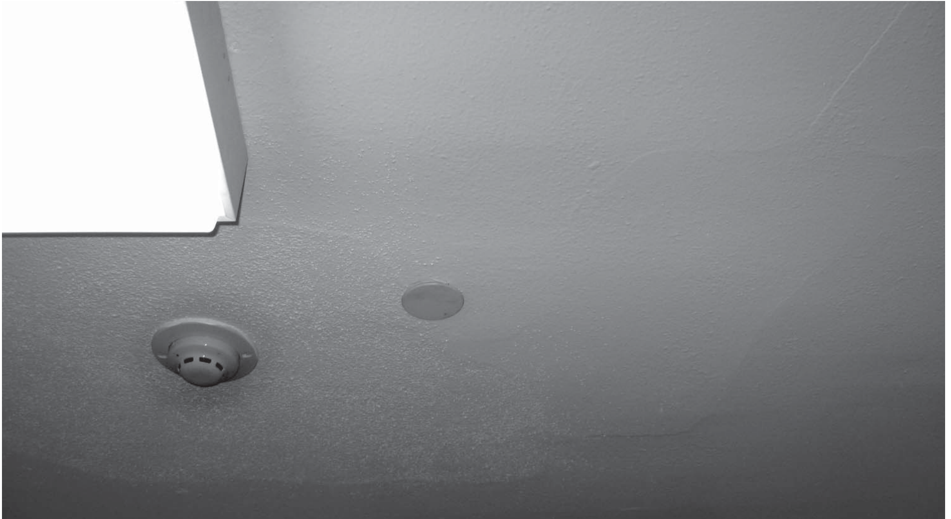
Figure 6.59: Ceiling of Room 6, note cracked and repaired plaster sections (Sommers, 2009)
