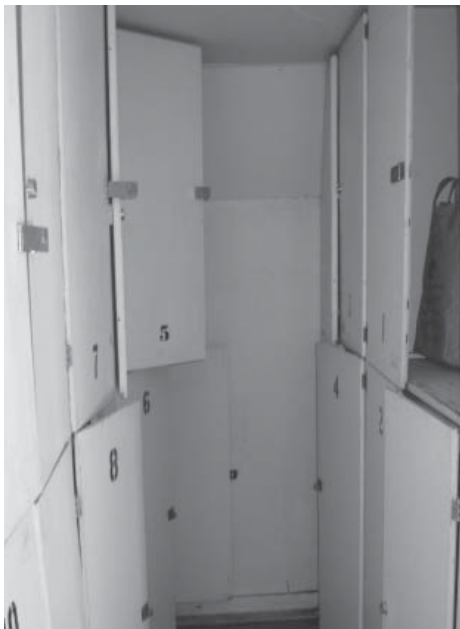
Figure 6.73: Above, garage attic roof structure, below, interior of storage room in garage building (Jaramillo, 2009)
