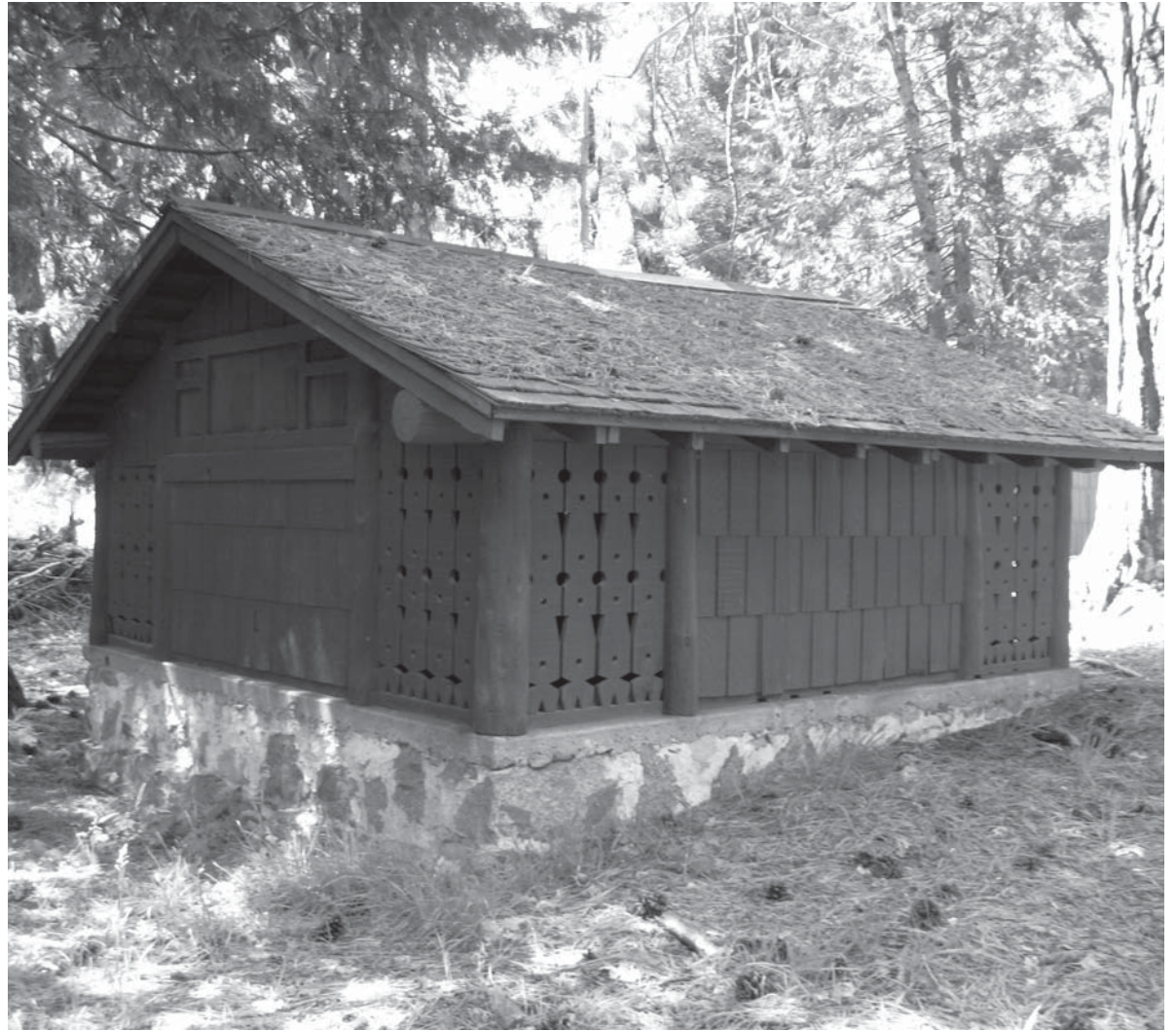
Figure 6.78: Northwest view of transformer building (Jaramillo, 2009)
