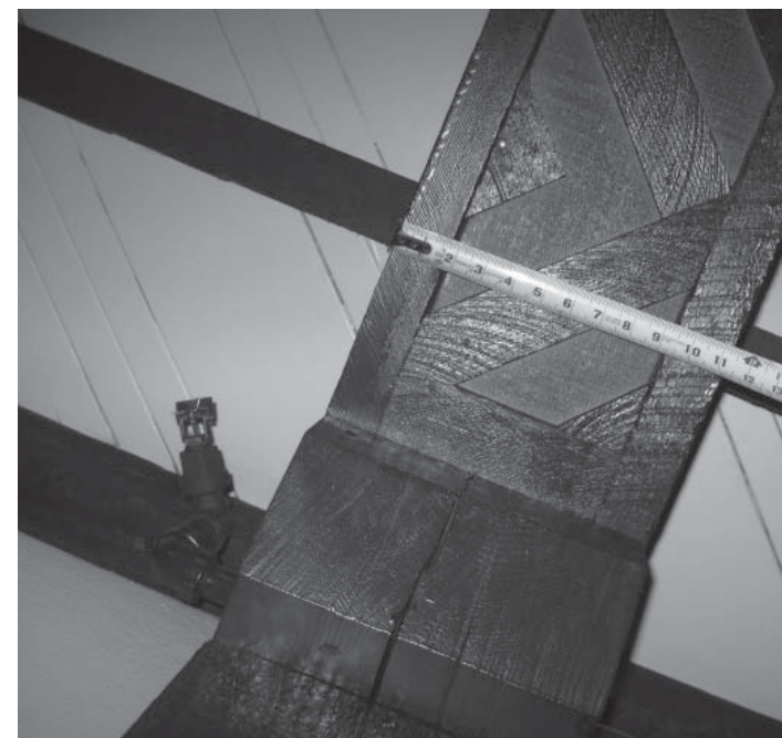
Figure 6.41: Detail view of builtup supporting beam with ceiling joists and added fire sprinkler head (Jaramillo, 2009)
