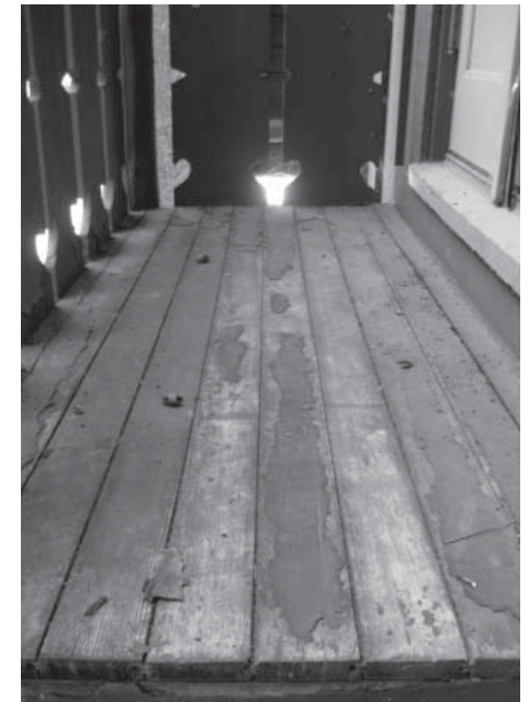
Figure 6.28: Above, damaged and racking balcony railing, above right, checked railing post infilled with silicone (detaching), below right, worn and deteriorated deck on north balcony/fire stair (Jaramillo, 2009)
