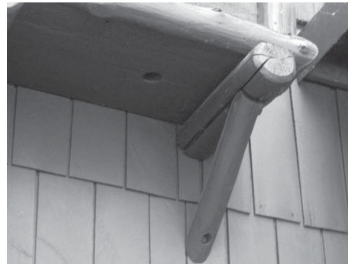
Figure 6.13: Above, water damaged log pilaster base, below, checked and split planter bracket. (Sommers, 2009)
