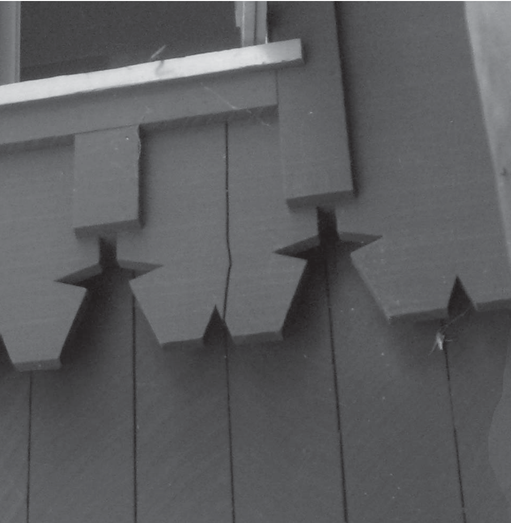
Figure 6.9: Split board on courtyard facade of clubhouse (Summers, 2009)
