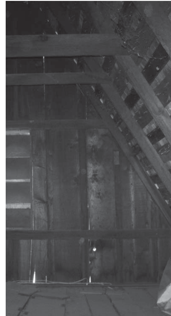
Figure 6.75: Attic interior of garage, note the vent to left of photograph (Jaramillo, 2009)
