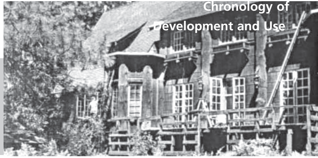
1953 Reconstruction of terrace - Note replacment of large cedar log columns
