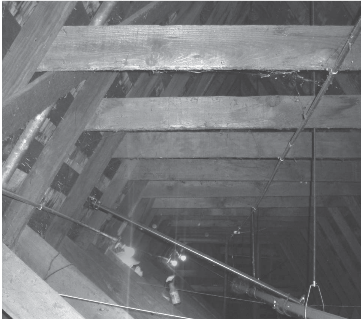
Figure 6.17: Attic view (Sommers, 2009)
