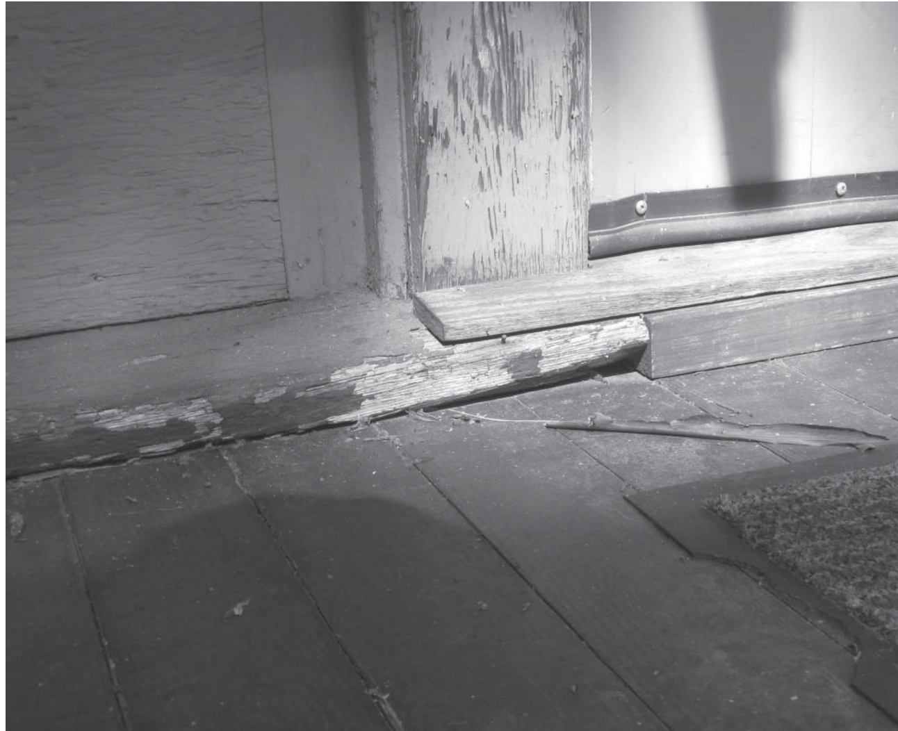
Figure 6.36: Damaged exterior sill on service entry. Note repair to sill and subsequent damage to it and surrounding trim. (Jaramillo, 2009)
