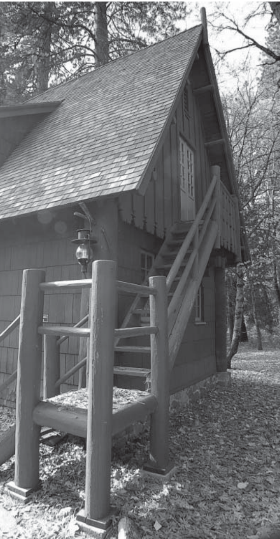
Figure 6.24: View of west fire staircase. Note lamp reproduction (Jaramillo, 2009)
