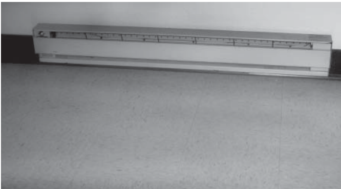
Figure 6.70: Above, electric heater in second floor shower room, below, baseboard heater in Dormitory B (Sommers, 2009)
