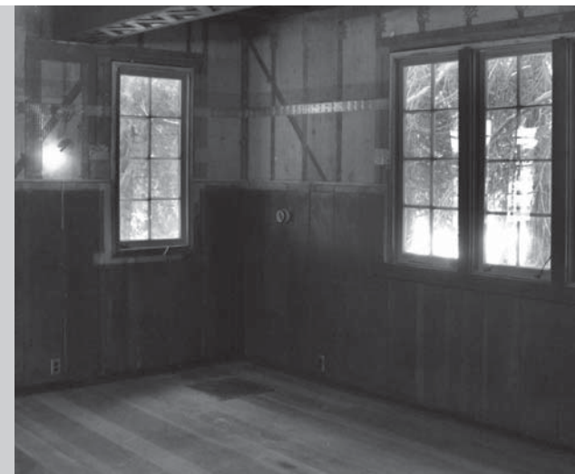
2008 Seismic upgrades throughout structure
