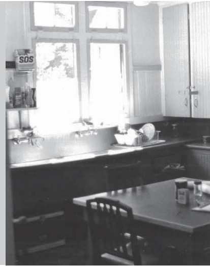
1972 Kitchen prior to renovation
