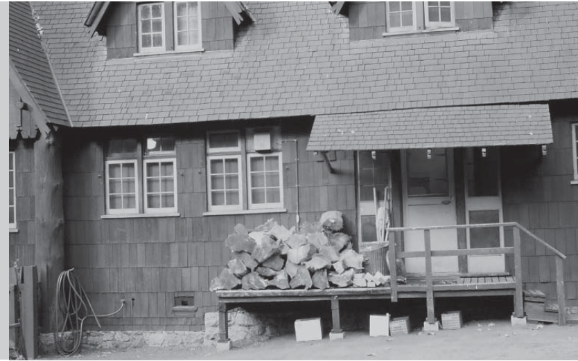
1970s Service porch with deterioration
