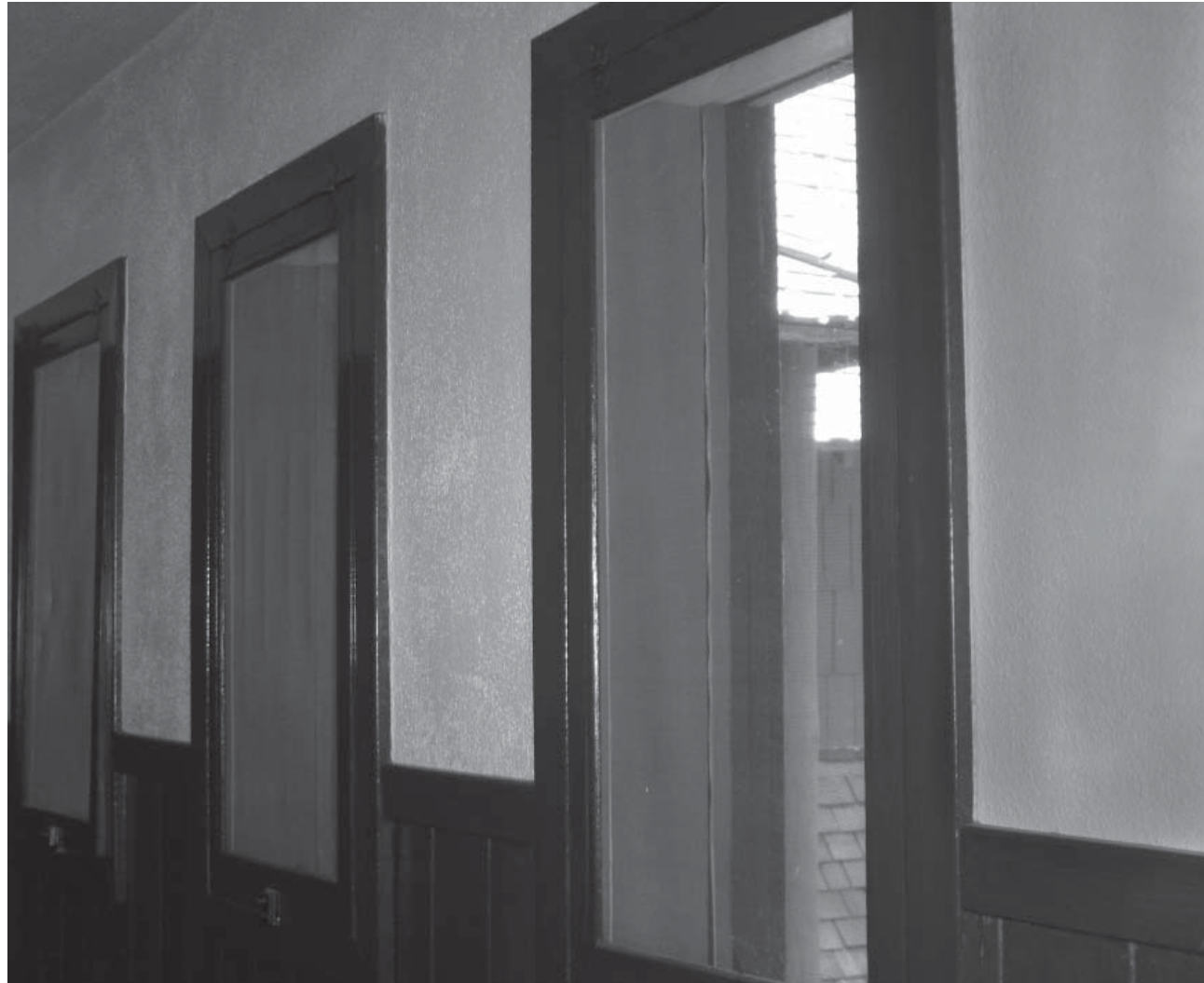
Figure 6.63: View of hallway windows on second floor, note simple trim details connecting with wainscoting (Jaramillo, 2010)
