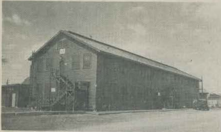
Outside view of new mess hall.
