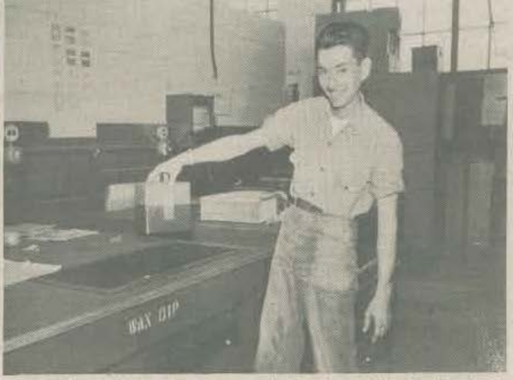
Dipping in wax to insure complete waterproofing as shown here by Louis Rottar, S/1c.
