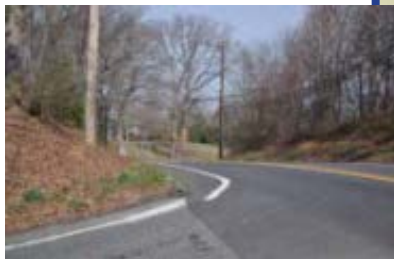
View north at Duley Station Road
