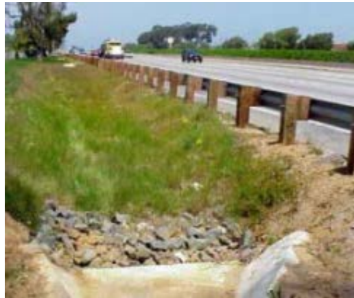
Example of an infiltration area associated with a highway in lieu of traditional drainage
