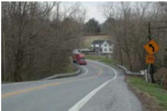
Use of a thicker edge line brings driver attention to the curve as an alternative to modifying the alignment to increase safety (Maryland Historic National Road)
