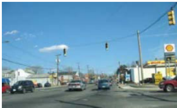
Portions of Bladensburg Road will be undergoing improvements as part of a “green highway” demonstration project
