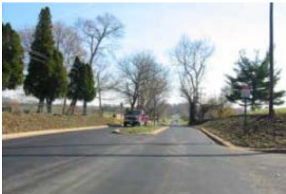
Splitter islands along U.S. Route 50 in Virginia were installed approaching Upperville as part of a national demonstration project for rural traffic calming
