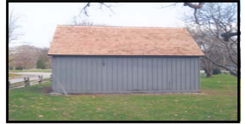
Roofing job completed
