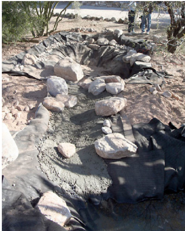
Backyard pond construction in progress
