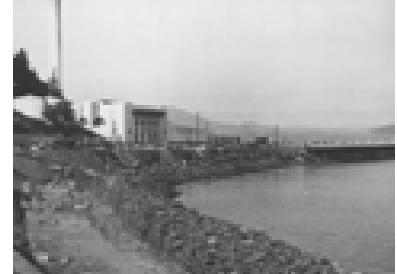
**Figure 9.** Large amounts of debris and rubble dumped along the shoreline of the cove were used to construct a crude seawall. (*San Francisco Maritime NHP, Historic Documents, Photograph Collection, P88-035.00033*)
