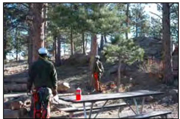
Hazard tree removal for visitor safety in Moraine Park Campground.
