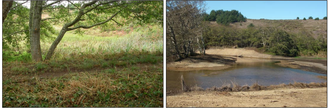
(Left: Before; Right: After) Removal of Muddy Hollow Dam (left) restored hydrologic connectivity between Muddy Hollow Creek and tidal flows (right).
