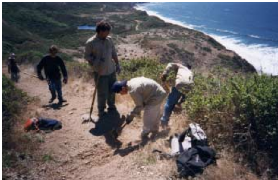
Youth Conservation Corps crews constructing water bars to reduce erosion.
