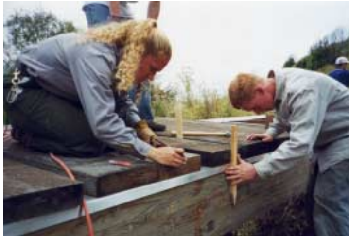
Crews repairing bridge walkway.
