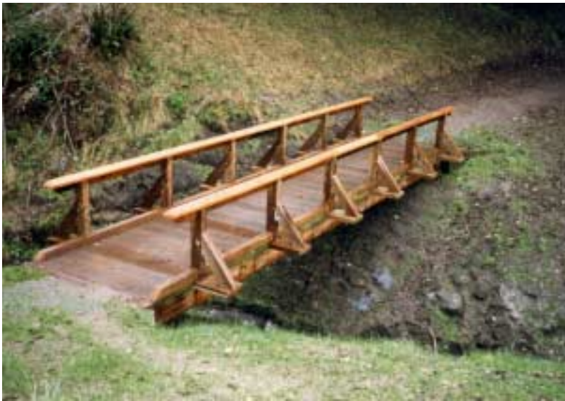
Standard rustic bridge used for creek crossings.
