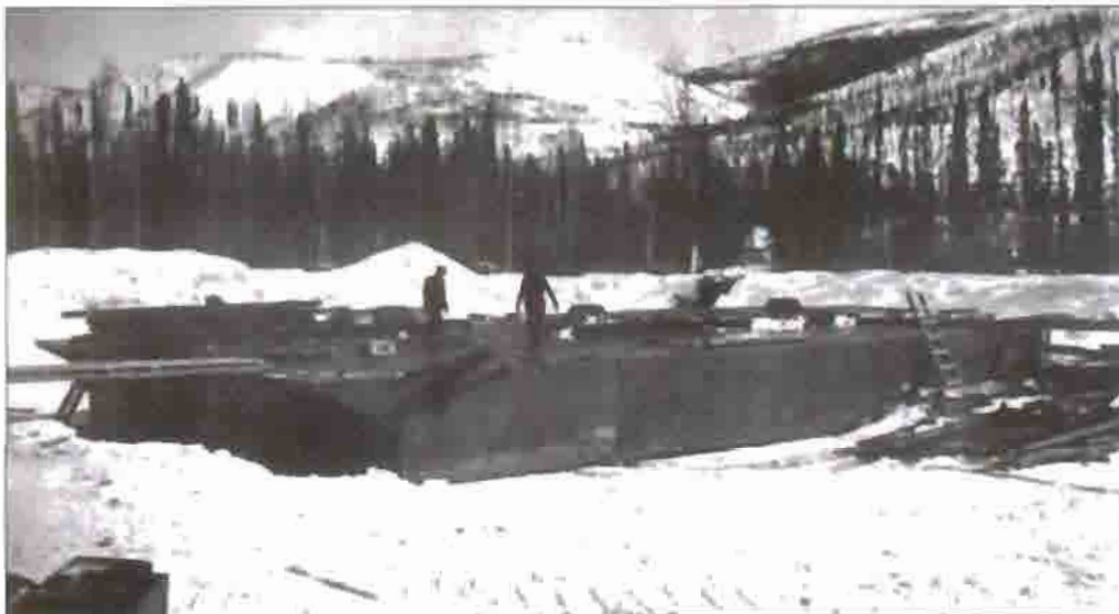
Metal "boxes" are assembled forming the pontoon hull are assembled on the frozen surface of the construction pond at Camp No. 1. NPS photo, Bill Lemm Collection.
