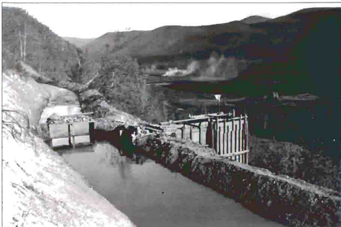
Penstock on the Coal Creek ditch. The penstock serves as a reservoir to hold water and build pressure or "head" for the water to force through the pipes used in the thawing and stripping process. The flag, visible on the penstock, indicated the level of the water to the crews working in the valley below. The main hydraulic ditch is visible running across the valley on the right, with a bridge supporting it across Coal Creek. Everett Hamman Collection, University of Alaska – Fairbanks, Rasmuson Library (Acc. #85-110-09).
