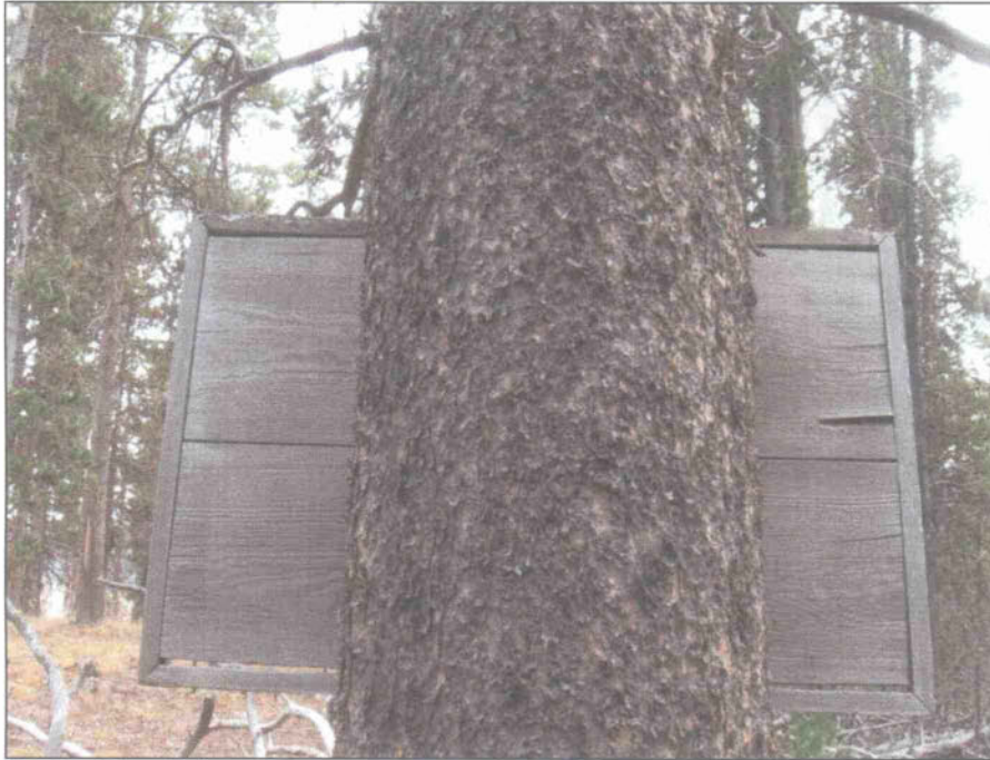
Back side of sign. Note center portion of sign consists of two 1" boards. Note also that the center boards have shrunk relative to the frame.
