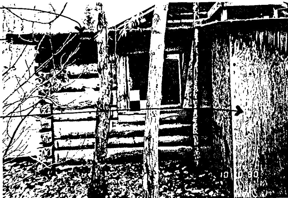
WEST ELEV - NW CORNER
