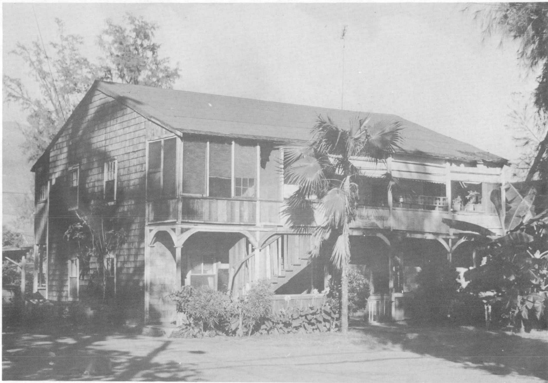
United States Marine Hospital, Lahaina, Maui; erected in 1843, this stone building is a relic of whaling days.
