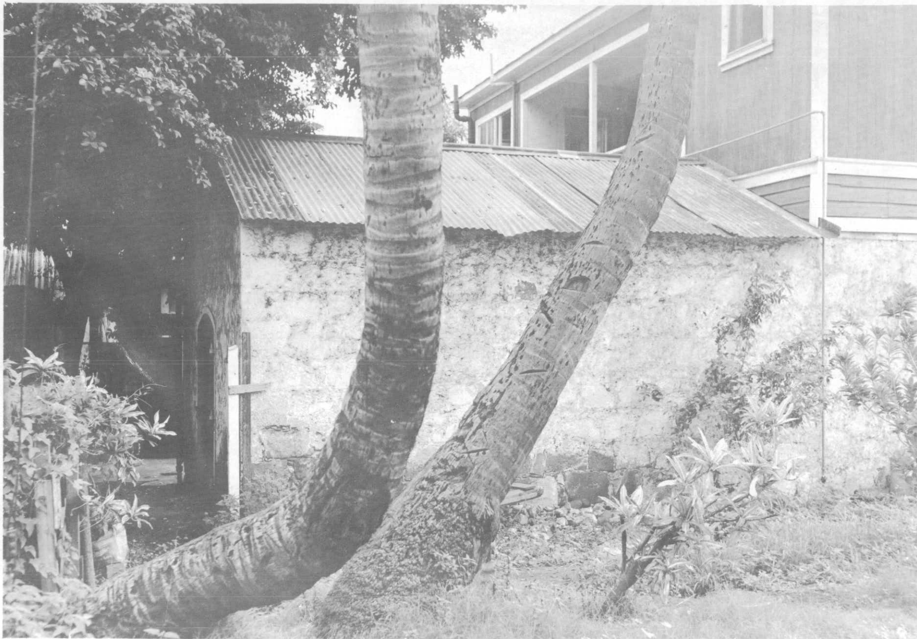
Old Spring House, Lahaina, Maui; built during the 1820's to enclose a spring from which Lahaina families and visiting ships obtained water.
