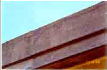
**Recommendation:** Remove spray-on roofing material. Rehabilitate concrete. Costs reflect both removal of roofing material and rehabilitation of 100% of surface area.
