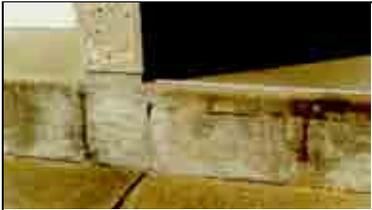
**Recommendation:** Conduct a thorough investigation to understand the cause of spalling conditions. Repair using sound preservation practices and concrete repair techniques. Costs reflect rehabilitation of 50% of surface area.
