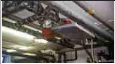
**Recommendation:** Replace with a new pump, including flexible pipe connectors and hanger rod at pump connections.
